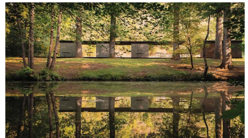
Bathing Pavilion in Olot, Spain by RCR Architects: This is a simple structure where the roof is supported by small banks which accommodate bathrooms and facilities for bathers. The roof spanning between them provides an external covered space. This is an example for the types of structures / welfare facilities that could be provided along the canal linear park for boat users.
