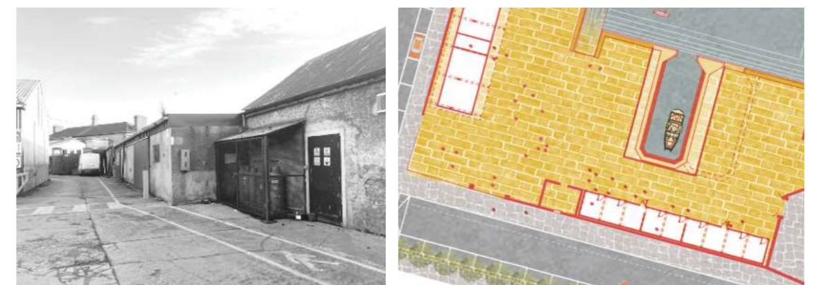
Existing condition with the carpentry workshops on the right and the Dry Dock to the left. The dimension between the carpentry workshop and Dry Dock is currently constricted. The new structure would alleviate this with its shallower depth.
