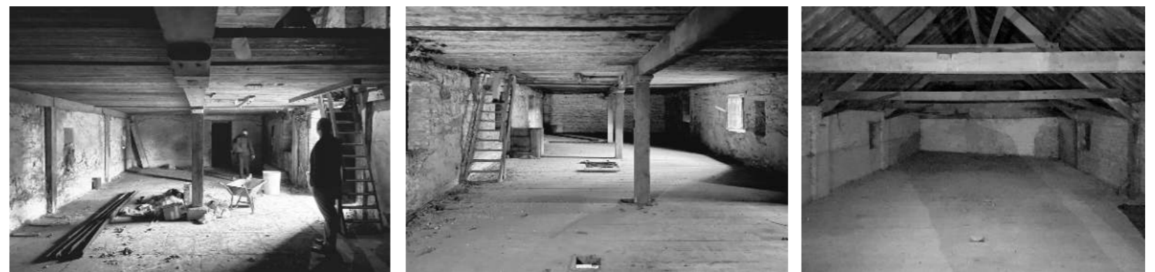
Ground, first and second floors (from left to right) at present in Young's Stores. Note the flagstone floors, timber central beam and columns and thick structural floorboards.
