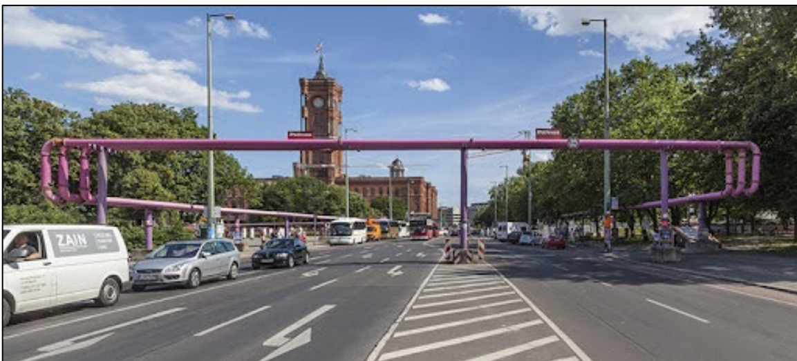
Figure 3-4: Elevated Pipe Installation (Berlin)
