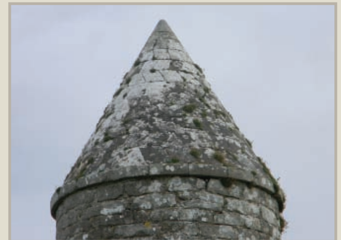
McCarthy's Tower; Clonmacnoise, today Note herringbone masonry pattern
