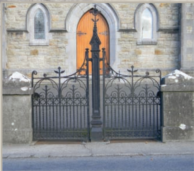
Ballinahown Church Gate Piers at road wall erected in 1904 by Egan's
