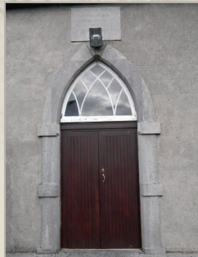
Door surround of former Roman Catholic Church, Shannonbridge (1858) in limestone
