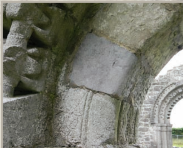
Repairs to Nuns' Church, Clonmacnoise undertaken in 1865
