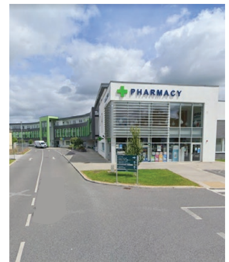
4 Primary Care Centre
