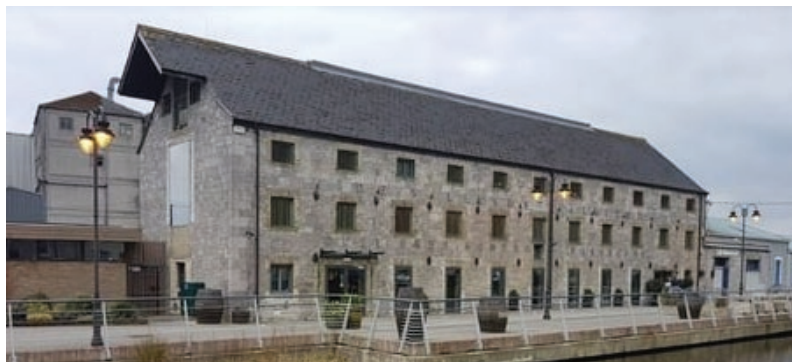
2 Former Tullamore Distillery (Protected Structure)
