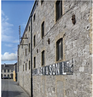
The Malthouse, Bridge Lane
