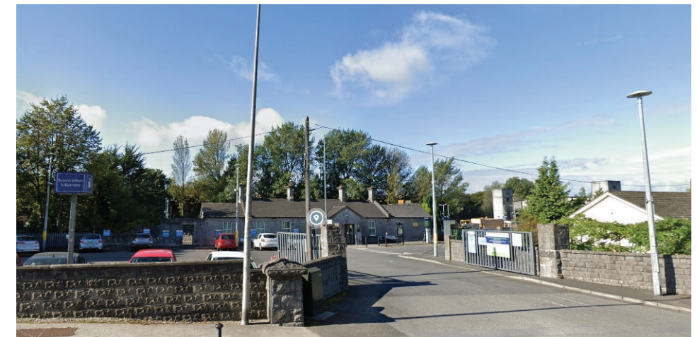
1 Tullamore Railway Station Entrance
