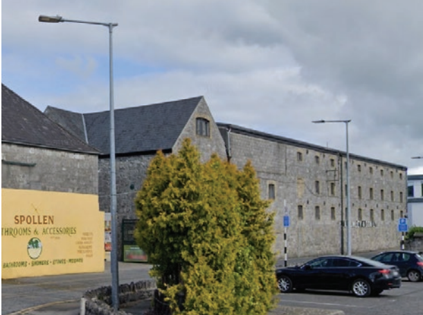
The Malthouse, Bridge Lane
