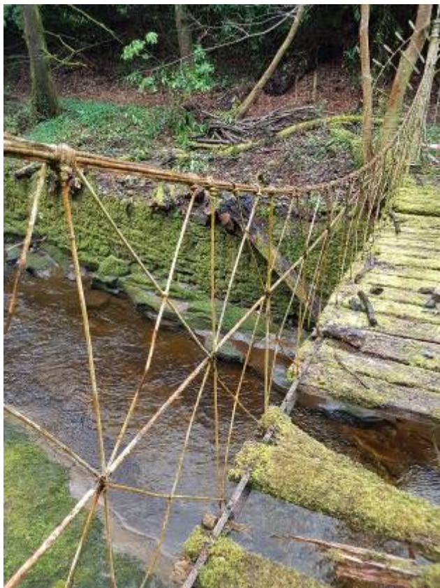
10. Wire hangers pass through 2 iron flats which support the oak floor. These are to be replaced with galvanised steel flats.
