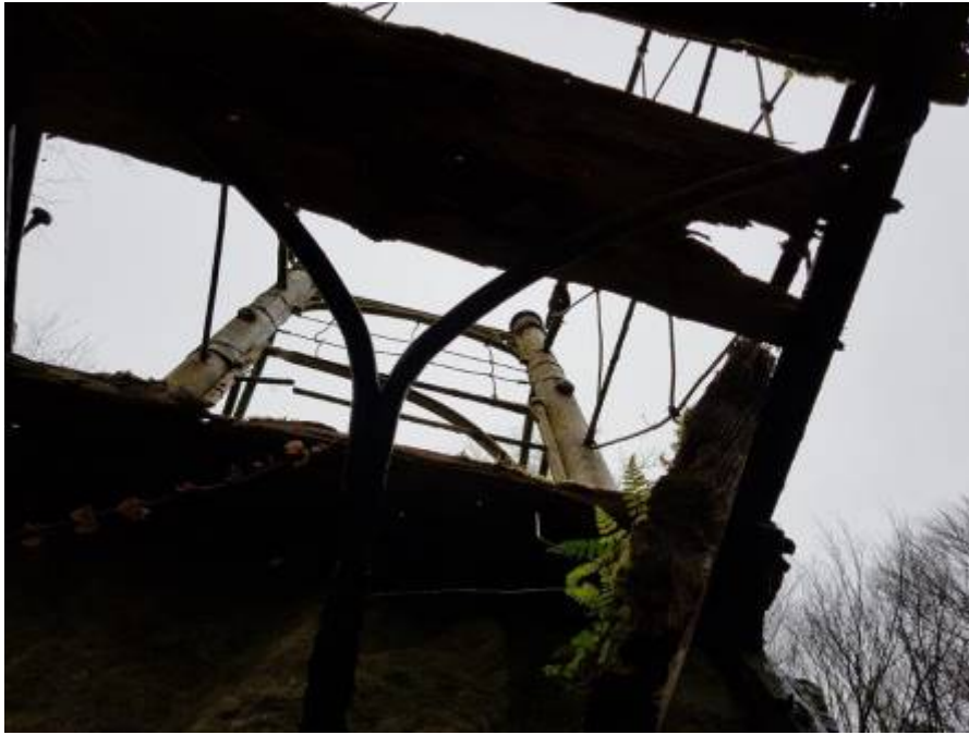
13. View of underside of bridge
