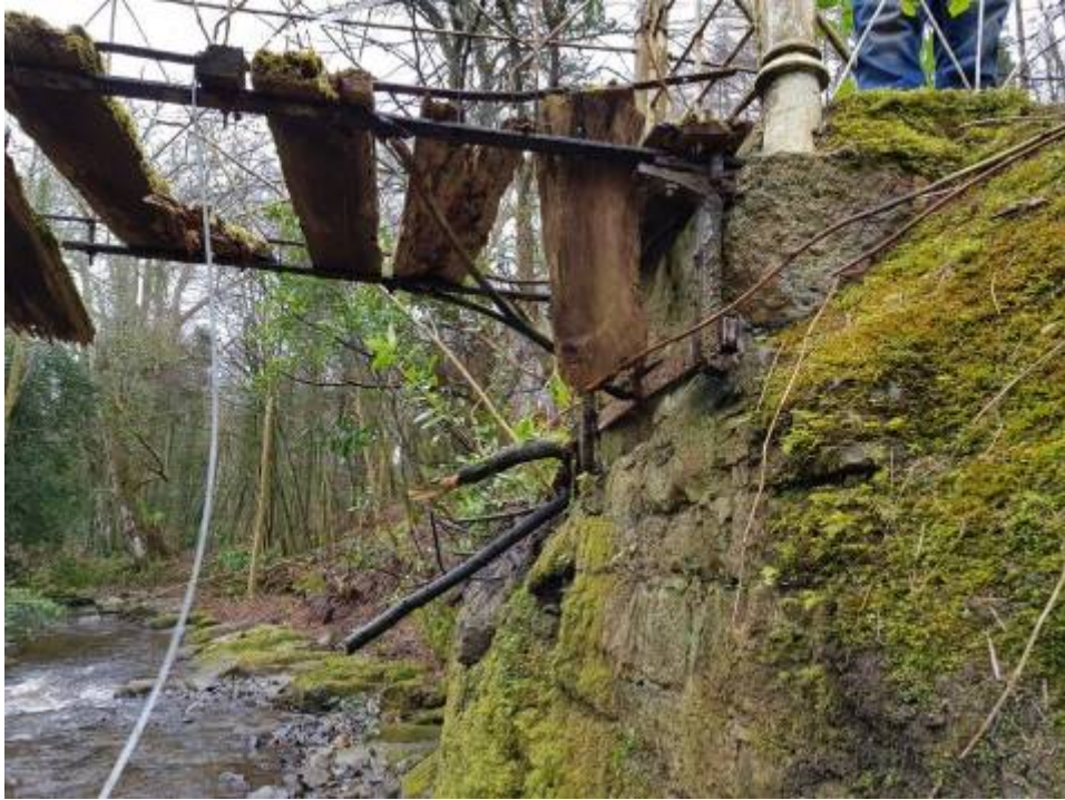
17. Detail of iron support to flats (not critical structurally)
