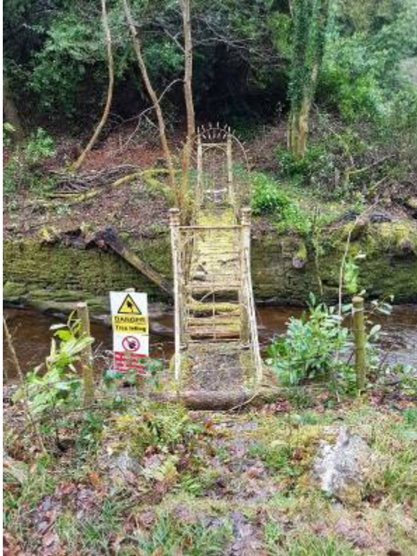
1. Approach to Suspension Bridge from Coillte side
