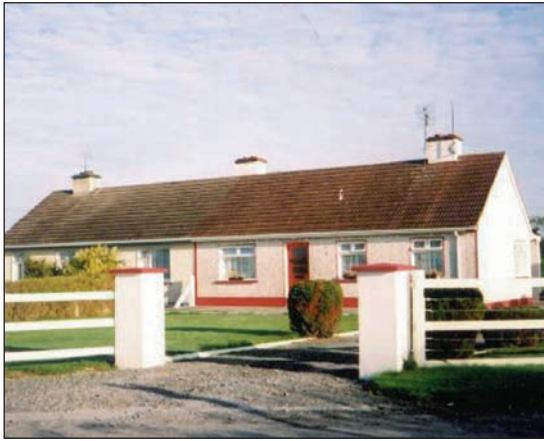
First of Local Authority houses built in 1954.
