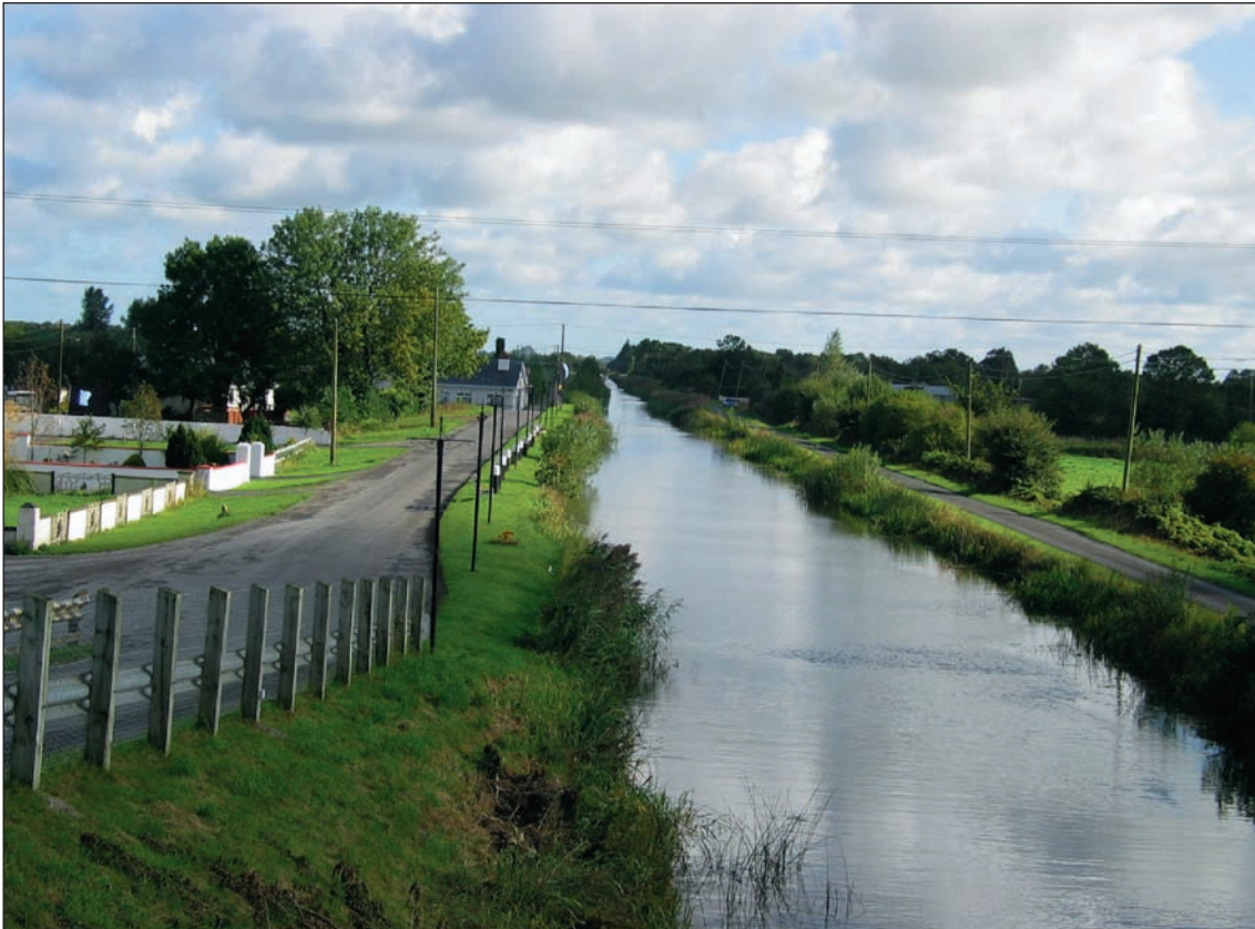
View of canal from Plunkett Bridge.
