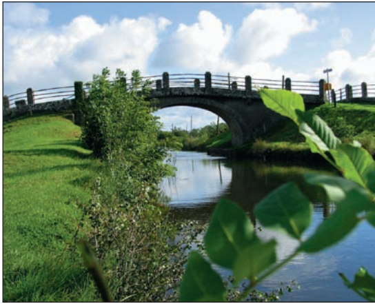
View of Plunkett Bridge.
