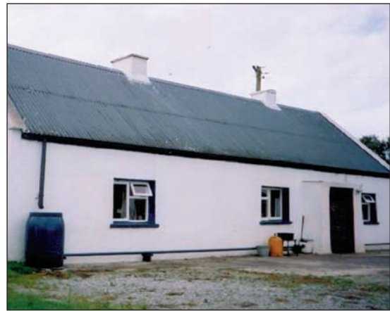
200 year old tin roofed house in VDS area.
