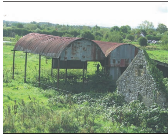
Remaining wall of house built of stone and Pullough brick.
