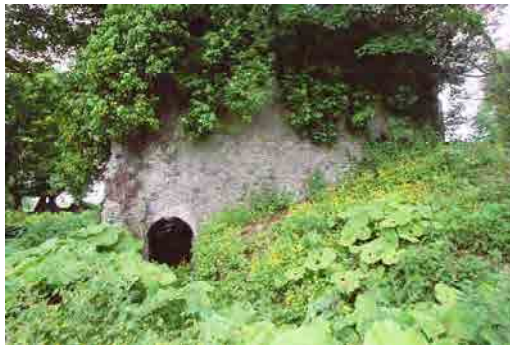
OFIAR-002-014_06 FWH 10/06/2003 Pond overflow tunnel under building.
