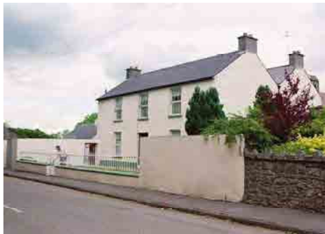
OFIAR-031-012_15 FWH 12/06/2004 Distillery House, from south-west.
