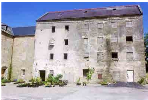
OFIAR-043-002_04 FWH 18/07/2003 South elevation of mill.
