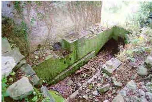
OFIAR-042-012_06 FWH 01/08/2003 Waterwheel pit at north end of grain/cloth mill.
