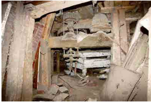
OFIAR-009-005_08 FWH 11/06/2003 Modern roller on ground floor.
