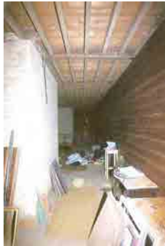
OFIAR-031-012_11 FWH 31/07/2003 Second floor of kiln. Note perforated tiles.
