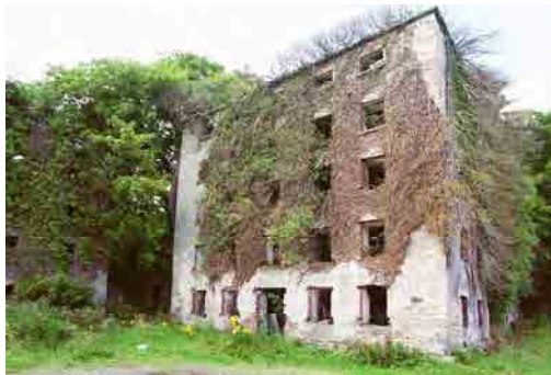
OFIAR-042-012_03 FWH 01/08/2003 Grain/cloth mill, from south-west.
