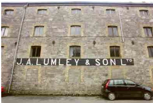
OFIAR-017-039_04 FWH 31/07/2003 Detail of east elevation of malt house 1.
