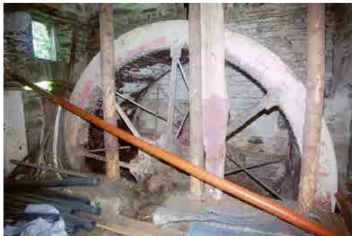
OFIAR-043-002_07 FWH 18/07/2003 Mill: waterwheel on ground floor of west bay.
