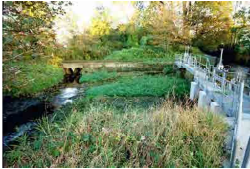
OFIAR-008-038_17 FWH 15/10/2003 Looking east along River Brosna. Headrace to Erry Mill on left bank (at right), and aqueduct from headrace on right bank (at left).
