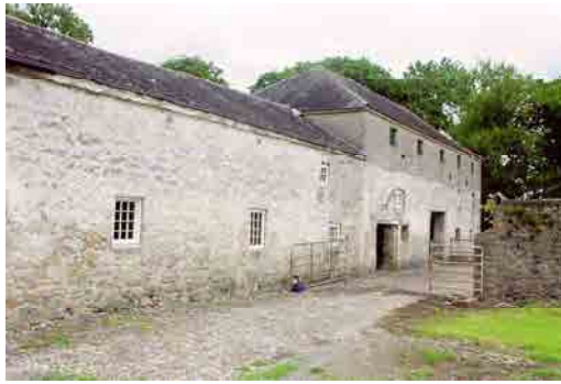
OFIAR-042-033_02 FWH 01/08/2003 Kiln (at centre), with three-storey granary to right, from south-west.
