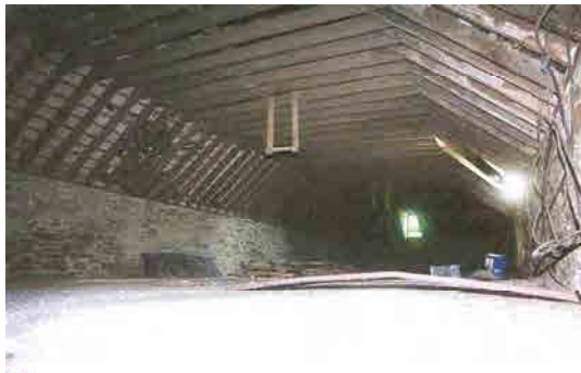
OFIAR-043-002_19 FWH 18/07/2003 Grain store: attic floor, looking north.
