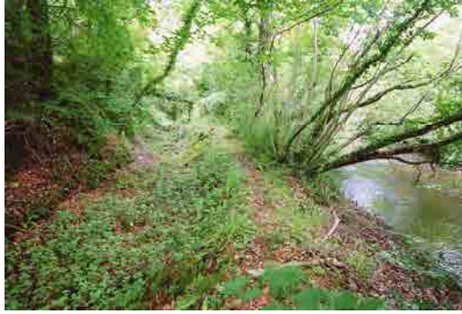
OFIAR-032-002_05 FWH 12/06/2003 Looking up waterwheel pit towards water intake end. Note semi-elliptical brick arch at far end.
