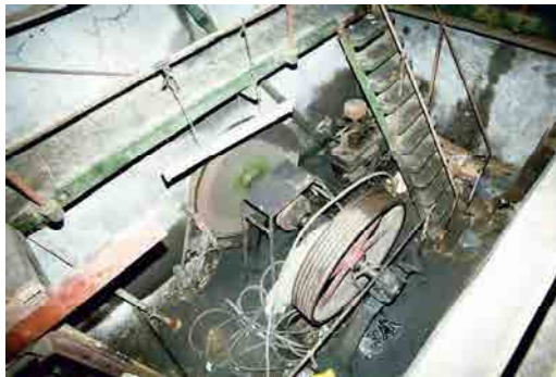
OFIAR-008-038_10 FWH 15/10/2003 Vee pulley at end of turbine lineshaft in basement of boiler/generator house.
