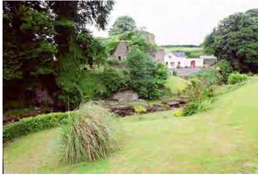
OFIAR-037-002_02 FWH 26/06/2003 Mill complex from east.
