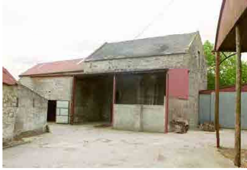
OFIAR-009-005_04 FWH 11/06/2003 Store and cascade drying room, from south.
