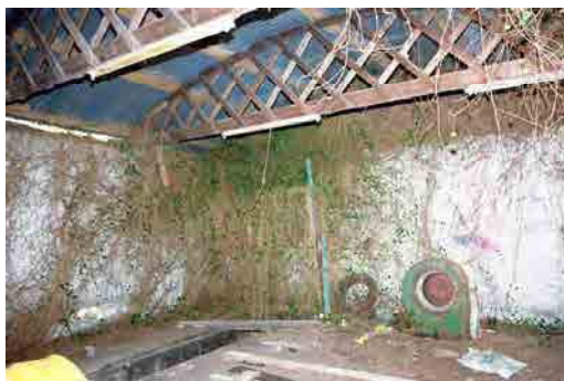
OFIAR-008-038_15 FWH 15/10/2003 Belfast truss room in shed.
