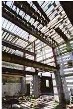
OFIAR-021-009_09 FWH 25/06/2003 Floor detailing in building 2 (maltings).
