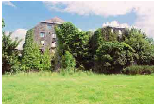
OFIAR-042-009_04 FWH 18/07/2003 General view from west.
