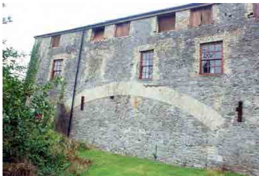
OFIAR-035-034_05 FWH 12/09/2003 West end of south elevation of south block.
