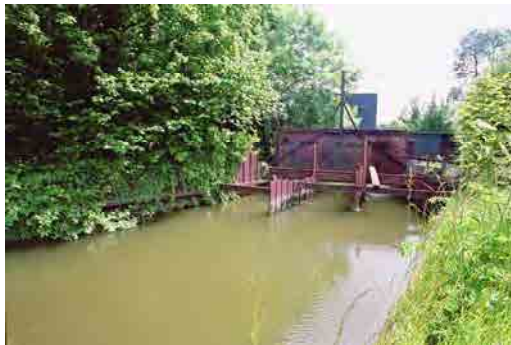
OFIAR-014-004_10 FWH 24/06/2003 Sluice gate emplacement above electricity station 2.
