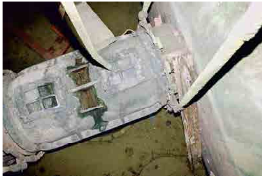
OFIAR-008-038_19 FWH 15/10/2003 Looking down into turbine emplacement. Note turbine guide vanes at right.
