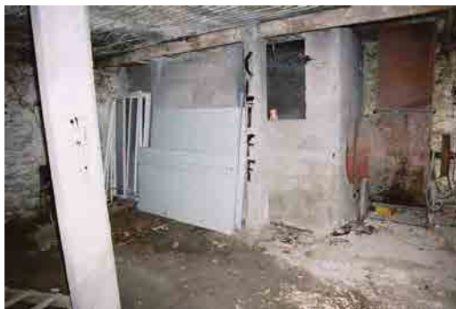
OFIAR-021-011_14 FWH 25/06/2003 Kiln (component 7): ground floor showing warm air intake duct.
