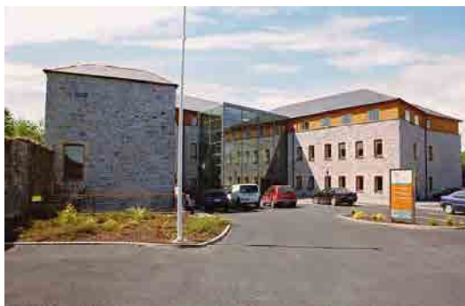
OFIAR-035-009_04 FWH 26/06/2003 Birr Technology Centre, from north. Waterwheel pit is on left gable.
