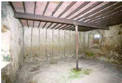
OFIAR-042-033_03 FWH 01/08/2003 Underside of kiln drying floor.
