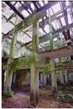
OFIAR-021-009_08 FWH 25/06/2003 Internal reinforced-concrete framework inside south section of building 1 (maltings).
