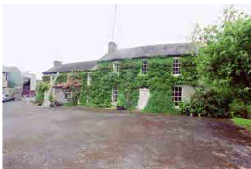
OFIAR-035-031_05 FWH 27/06/2003 Mill house, from south-east.
