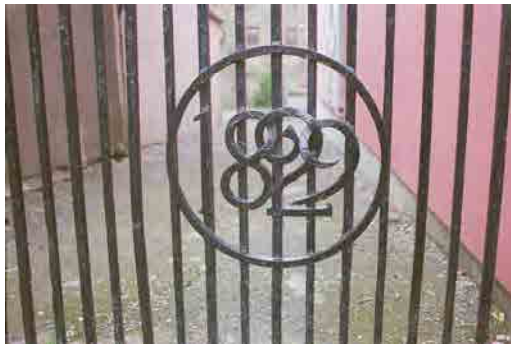
OFIAR-017-090_06 FWH 16/07/2003 1822 detailing on Patrick Street gates.
