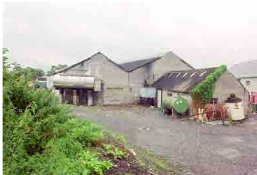
OFIAR-012-027_03 FWH 31/07/2003 Yard buildings, from north.
