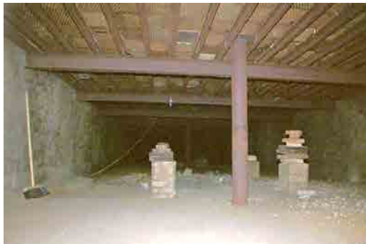
OFIAR-031-012_11 FWH 31/07/2003 Second floor of kiln. Note perforated tiles.
