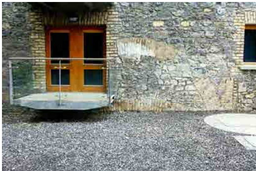
OFIAR-035-046_08 FWH 12/09/2003 Infilled archway on south gable of grain store.
