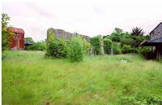
OFIAR-008-054_09 FWH 23/06/2003 Rubble wall to east of mill, from north-west.
