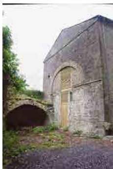
OFIAR-035-046_03 FWH 27/06/2003 South gable of former brewery and kiln remains.
