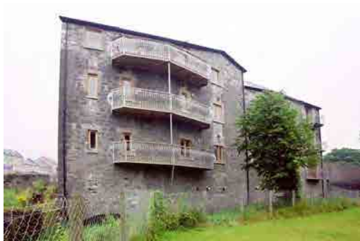
OFIAR-017-038_04 FWH 16/07/2003 South elevation, from south-west.
