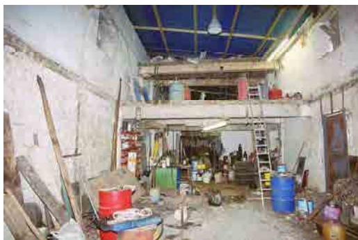
OFIAR-031-005_12 FWH 01/08/2003 Refurbished interior of store, to north.
