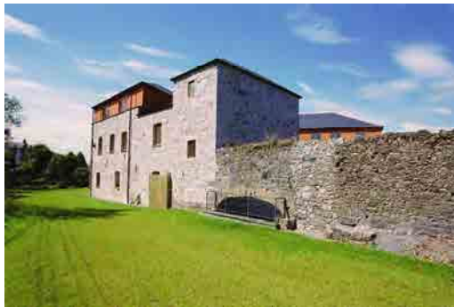
OFIAR-035-009_03 FWH 26/06/2003 Birr Technology Centre, from north-east. Note headrace intake arch.
