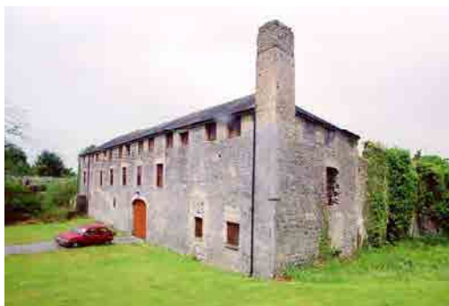
OFIAR-035-034_04 FWH 27/06/2003 South block, from south-east.
