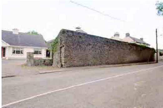
OFIAR-031-012_14 FWH 12/06/2004 Rubble boundary wall along west side of site.
