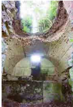
OFIAR-042-030_03 FWH 01/08/2003 Barrel vaulted return.
