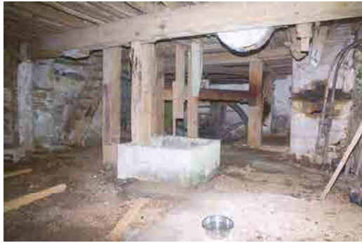
OFIAR-043-002_10 FWH 18/07/2003 Mill: Pitwheel, wallower and upright shaft on ground floor of east bay.
