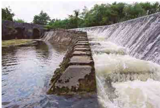
OFIAR-014-004_14 FWH 24/06/2003 Weir and fish pass, from west. Note inscribed stone at top of pass.
