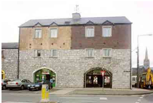
OFIAR-017-049_06 FWH 31/07/2003 North end of east elevation, from east.
