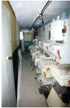
OFIAR-008-038_26 FWH 15/10/2003 First floor of east section of mill, looking south (former roller floor). Note duct trunking in ceiling.
