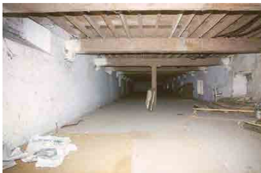
OFIAR-031-012_04 FWH 31/07/2003 Looking east across first floor of malting.
