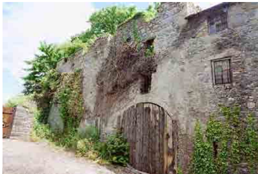
OFIAR-031-007_04 FWH 12/06/2003 West elevation of store, from south-west. Note tailrace arch (boarded over).
