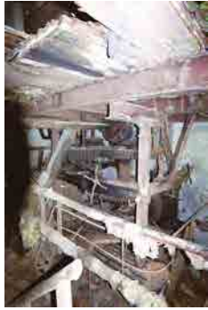
OFIAR-017-036_09 FWH 16/07/2003 Building 2: triple-throw pump on ground floor.
