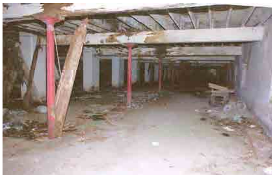
OFIAR-017-064_04 FWH 16/07/2003 Looking east along ground floor of malt house. Note timber transoms.
