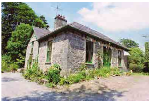
OFIAR-014-004_06 FWH 24/06/2003 Mill house, from south-west.
