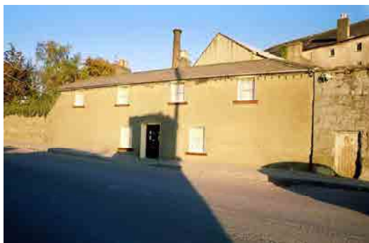
OFIAR-008-038_07 FWH 15/10/2003 Mill house 1 fronting Bridge St, from west.
