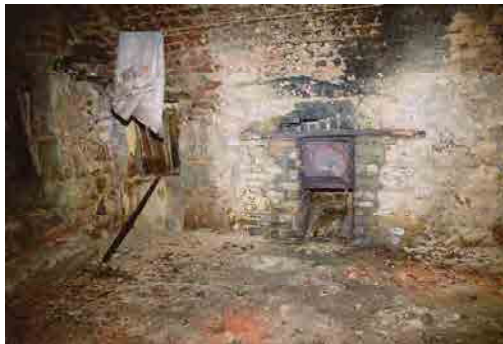
OFIAR-009-006_13 FWH 11/06/2003 Kiln: right-hand kiln furnace.
