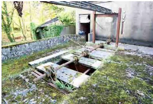
OFIAR-008-038_19 FWH 15/10/2003 Looking down into turbine emplacement. Note turbine guide vanes at right.
