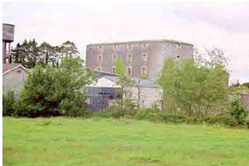
OFIAR-031-005_04 FWH 12/06/2003 General view of complex from south-west.
