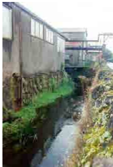
OFIAR-008-028_04 FWH 11/09/2003 South elevation of canteen and tailrace, from west.
