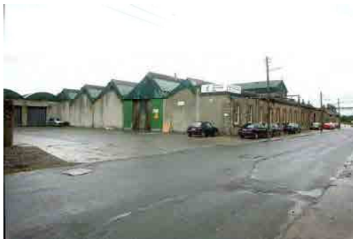
OFIAR-008-028_09 FWH 11/09/2003 Spinning factory on south side of road, from east.
