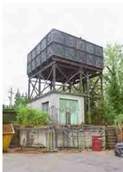
OFIAR-017-085_09 FWH 16/07/2003 Water tank at south end of site, from north.
