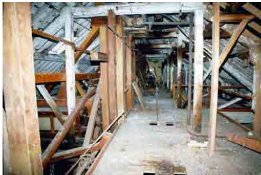
OFIAR-008-038_31 FWH 15/10/2003 Roofspace gallery, looking south.
