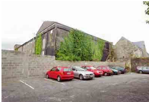
OFIAR-017-039_12 FWH 31/07/2003 General view of site from south-west. Malt house 2 at left.
