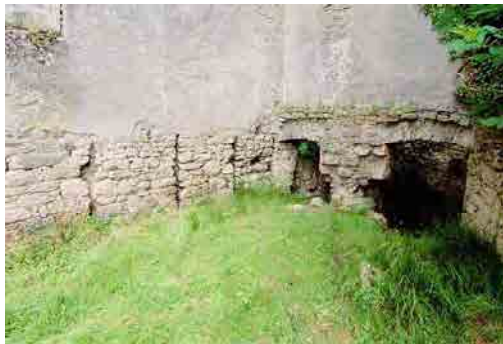
OFIAR-042-030_04 FWH 01/08/2003 Headrace intake on back wall of mill.
