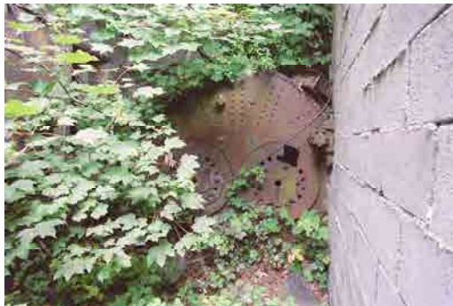
OFIAR-017-036_15 FWH 16/07/2003 Building 4: exposed end of boiler on SW elevation.
