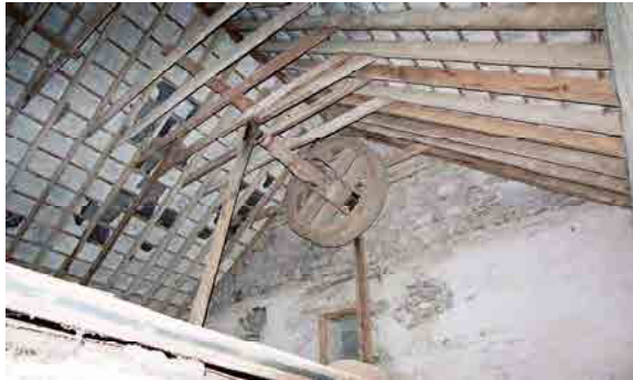
OFIAR-011-021_04 FWH 13/06/2003 Sack hoist on top floor of mill.
