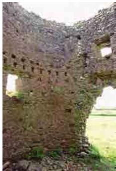
OFIAR-029-008_03 FWH 25/06/2003 Interior, showing floor beam sockets.
