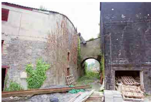
OFIAR-017-064_03 FWH 16/07/2003 Link between malt house and kiln, from north.
