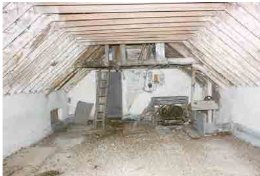
OFIAR-031-012_07 FWH 31/07/2003 East end of top floor of malting.
