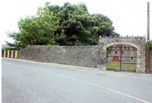
OFIAR-035-034_09 FWH 12/09/2003 Boundary and entrance on main road, from south.
