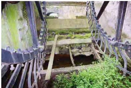
OFIAR-017-038_08 FWH 16/07/2003 Curved metal apron at back of waterwheel.
