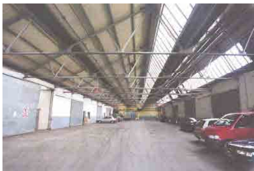
OFIAR-017-085_08 FWH 16/07/2003 Interior of mill.
