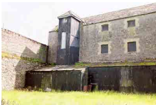
OFIAR-031-012_03 FWH 12/06/2004 Loading bay at east end of north elevation.
