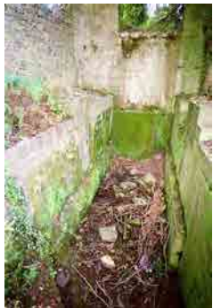
OFIAR-042-012_07 FWH 01/08/2003 Waterwheel pit at north end of grain/cloth mill.
