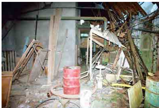
OFIAR-008-038_12 FWH 15/10/2003 Interior of south bay of boiler house.
