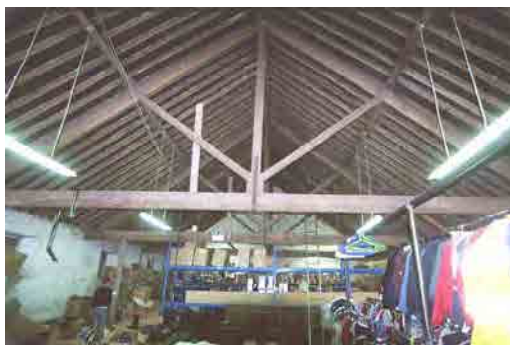
OFIAR-034-008_03 FWH 13/06/2003 Original roof trusses.
