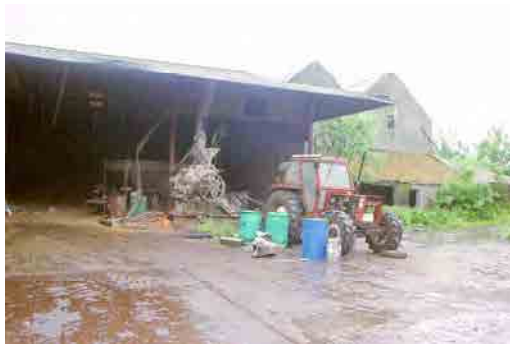
OFIAR-016-002_11 FWH 09/06/2003 Modern tractor-driven roller mill, from south.
