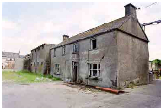
OFIAR-021-011_10 FWH 25/06/2003 Office (component 4), from south-west.
