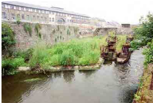
OFIAR-017-038_05 FWH 16/07/2003 Overgrown weir, from south-west.
