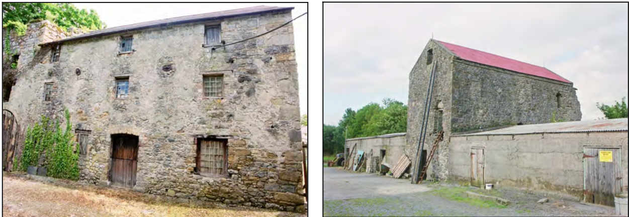
Fig 7.7a (left) Ballyboy Mill is now a domestic store (031-007.1). Fig 7.7b (right) Clonlisik Mill is now a farm outbuilding (045-105). Such converted buildings often have corrugated metal roofs in place of the original slate ones.
