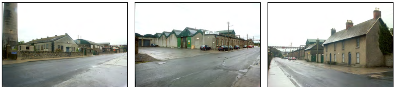
Fig 4.6 Clashawaun Jute Works (008-028). Top : OS six-inch map showing extent of works, 1910. Bottom left : Buildings along north side of road. The chimney at left is of mass concrete and dates from 1884. Bottom middle : Weaving sheds along south side of road. Bottom right : Houses on south side of road at west end of site.
