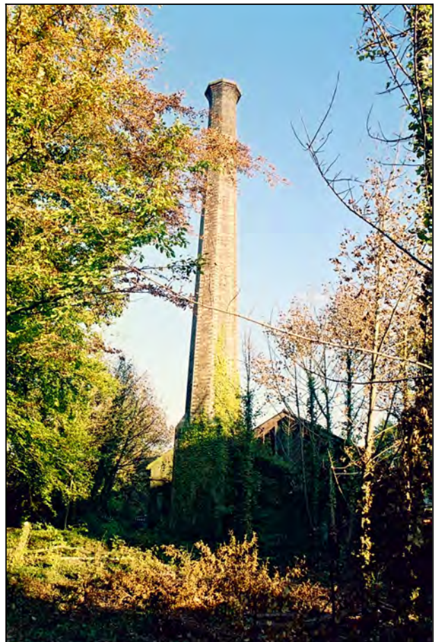
Fig 2.11 Brick steam engine chimney at Erry Mill (008-038).
