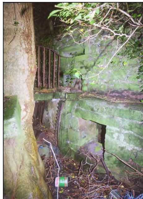
Fig 5.2 Waterwheel pit at the former mill in Charleville Demesne (16-031).
