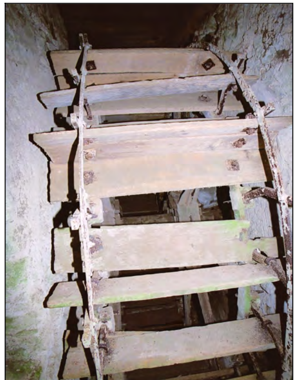
Fig 2.7 Paddle waterwheels. Top left: Schematic diagram of operation. Above: Paddle wheel at Belmont Corn Mill (014-004). Left: Skeletal frame of paddle wheel at Tullamore Mill (017-038).
