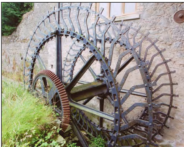
Fig 2.7 Paddle waterwheels. Top left: Schematic diagram of operation. Above: Paddle wheel at Belmont Corn Mill (014-004). Left: Skeletal frame of paddle wheel at Tullamore Mill (017-038).
