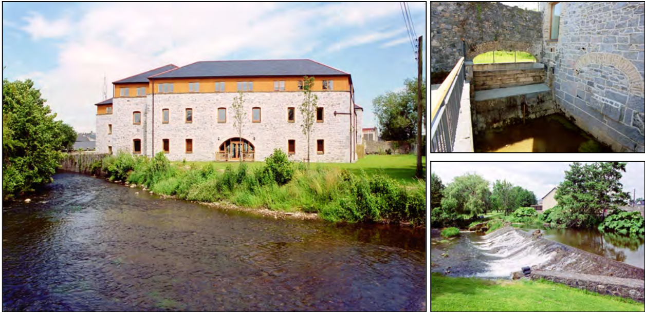
Fig 7.6 Birr Technology Park (035-009). Above: River elevation of partly rebuilt mill with new top floor. Top right: External waterwheel pit. Bottom right: Weir at start of headrace at Oxmanstown Bridge.
