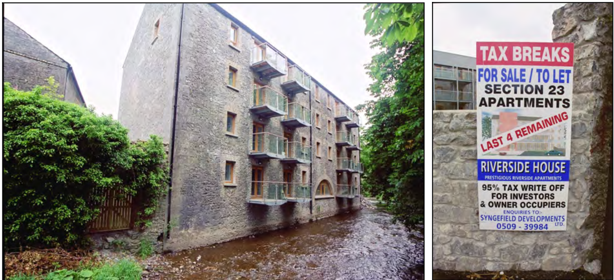
Fig 7.16 The apartments at the former Elmgrove Mill, now Riverside House (035-046).
