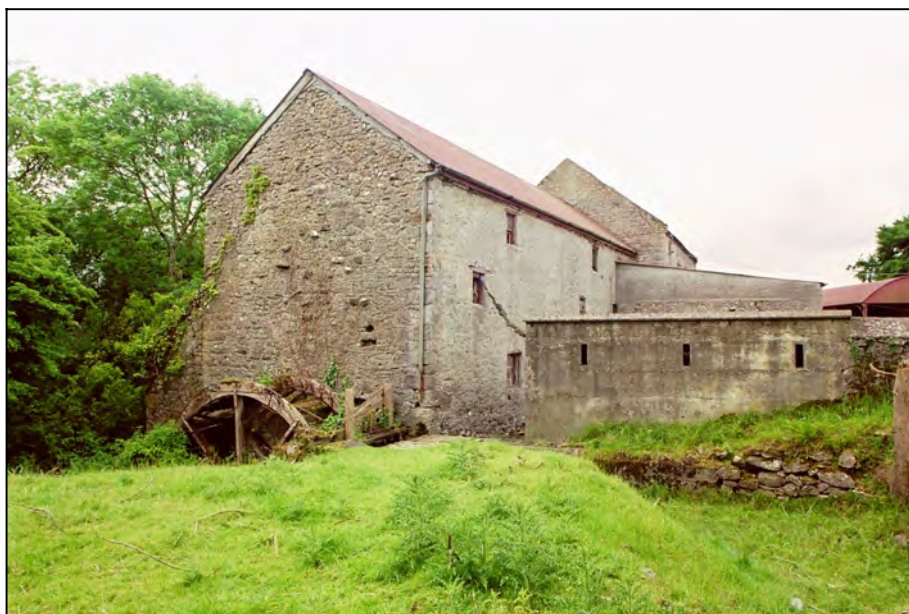
Fig 2.2 Acantha Corn Mill, north of Tullamore, a typical water-powered grain mill (009-005).
