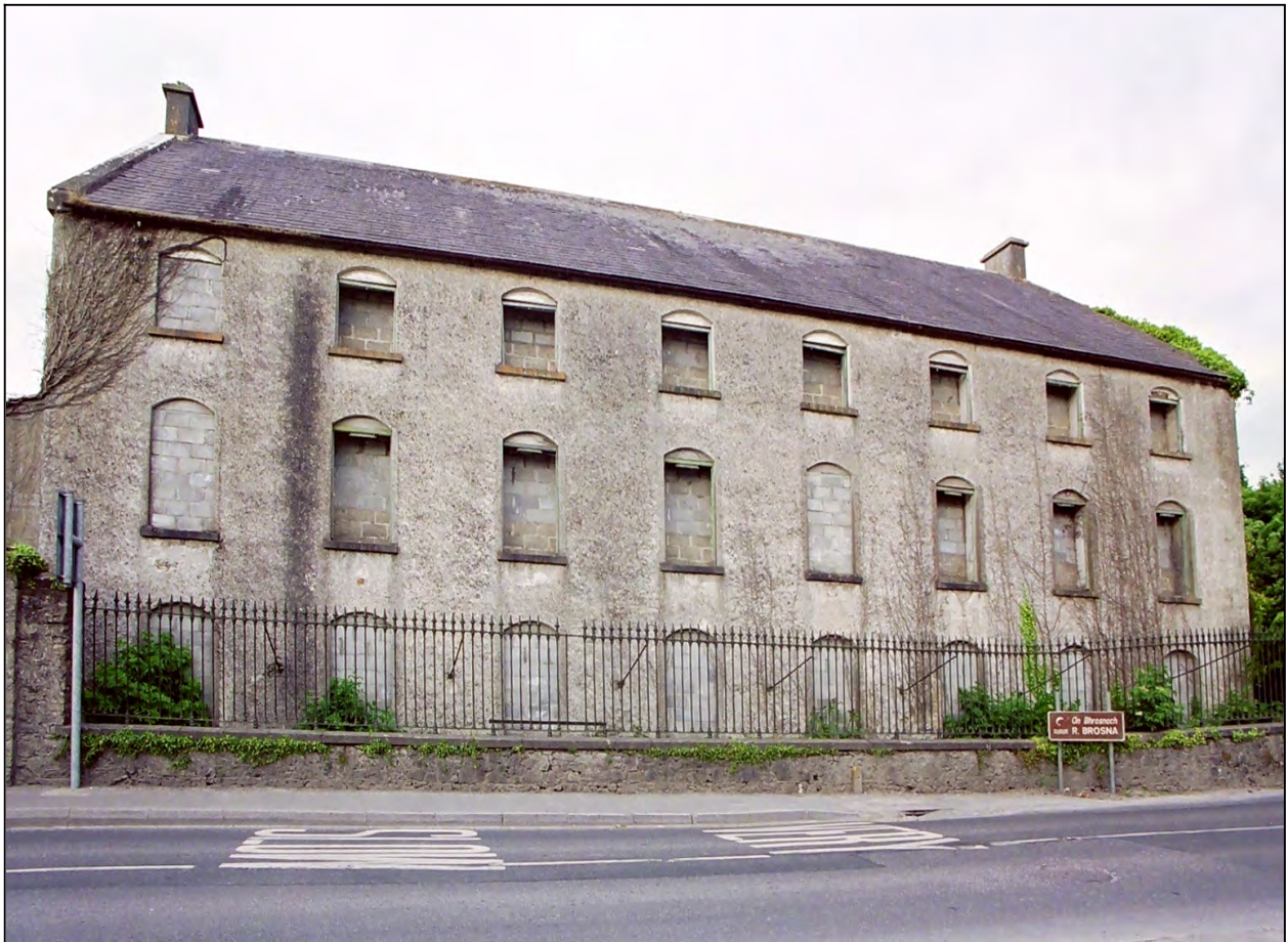
Fig 4.7 Cotton factory on outskirts of Clara (008-054), now disused.
