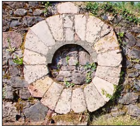
Fig 2.14a (far left) One-step shelling stone at Cappy- donnell Little Mill (002-006).
