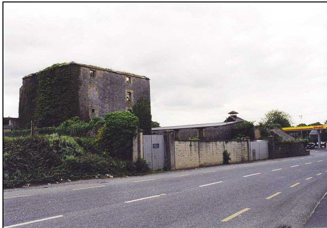
Photo 9 Ruinous Mill Buildings on the N52 Approach from Tullamore.
