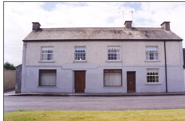
Photo 29 Former Shop in Use as a Private Residence
