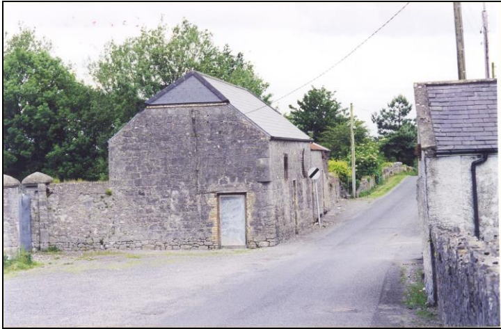
Photo 14 Secondary Route Directly off the North of Main Street
