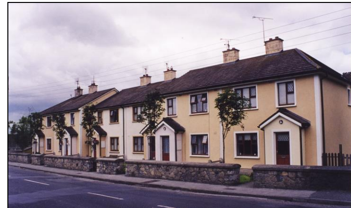
Photo 10 New Housing Development on Bridge Street
