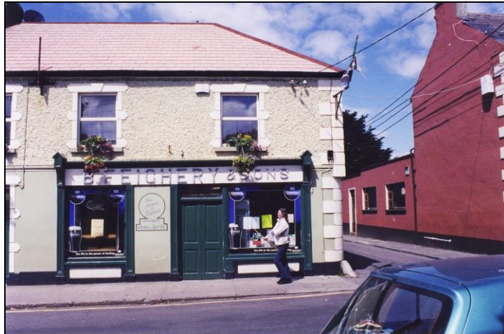
Photo 20 Building Edges Set out a Corner and Road Junction
