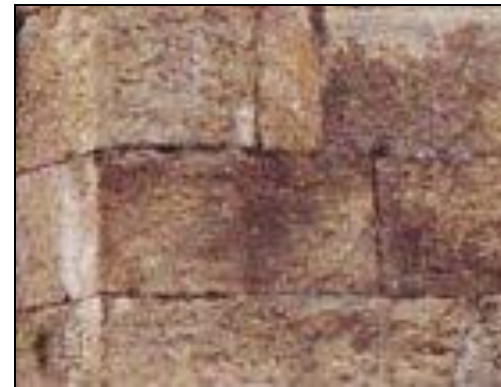
Photo27 Rubble Stone as Exposed by the Removal of a Finishing Plaster / Render.
