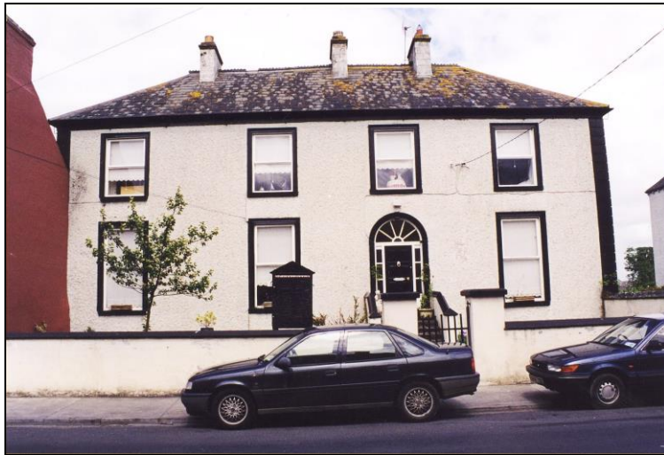
Photo 28 Attractive Building With Hipped Roof, Adjacent to the Convent, Main Street
