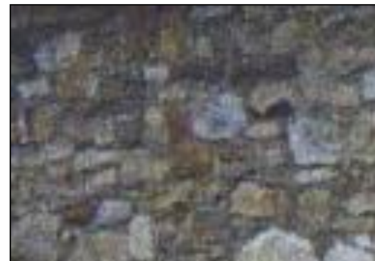
Photo27 Rubble Stone as Exposed by the Removal of a Finishing Plaster / Render.
