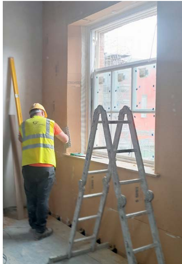
Figure 51: Woodfibre insulation board being prepared prior to application of finish coat
