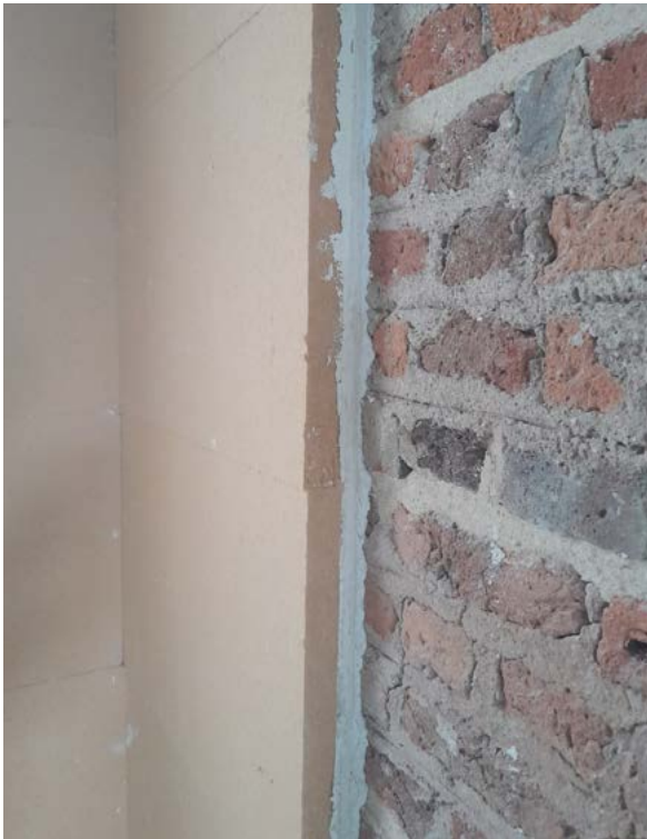
Figure 55: Build-up of lime mortar to level uneven surface prior to application of woodfibre board
