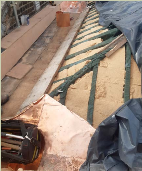
Figure 33: Wood-fibre insulating sarking board being applied between the rafters at roof level. (Image courtesy of OPW)
