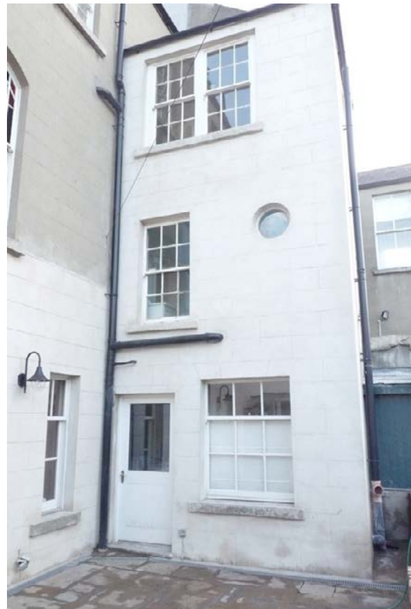
Figure 25: The same building with drainpipe leak fixed and the cement render replaced with a traditional moisture-permeable lime render. Note the addition of a channel drain, which helps to lower the ground moisture level close to the wall
