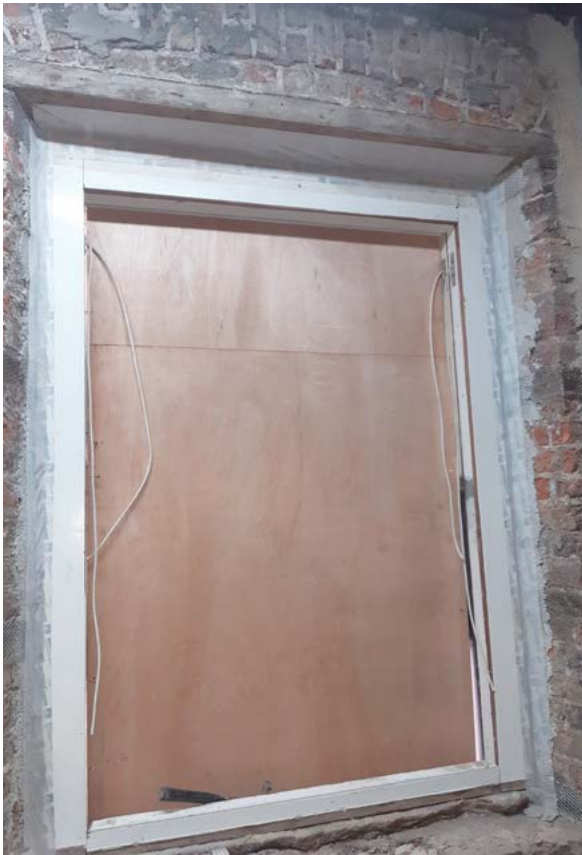
Figure 50: Tape to sash frame prior to application of IWI to ensure an airtight fit (Photograph by Con Brogan for OPW)
