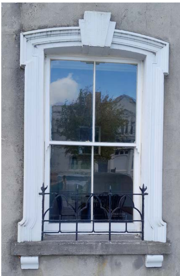
Figure 27: Timber sash window with some original glass panes
