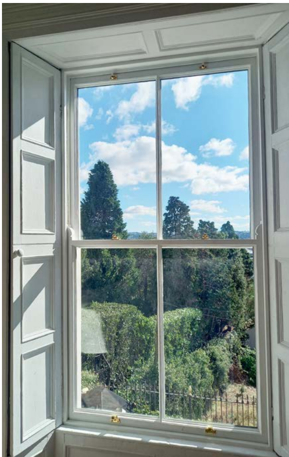
Figure 45: Two-over-two pane timber sash window
