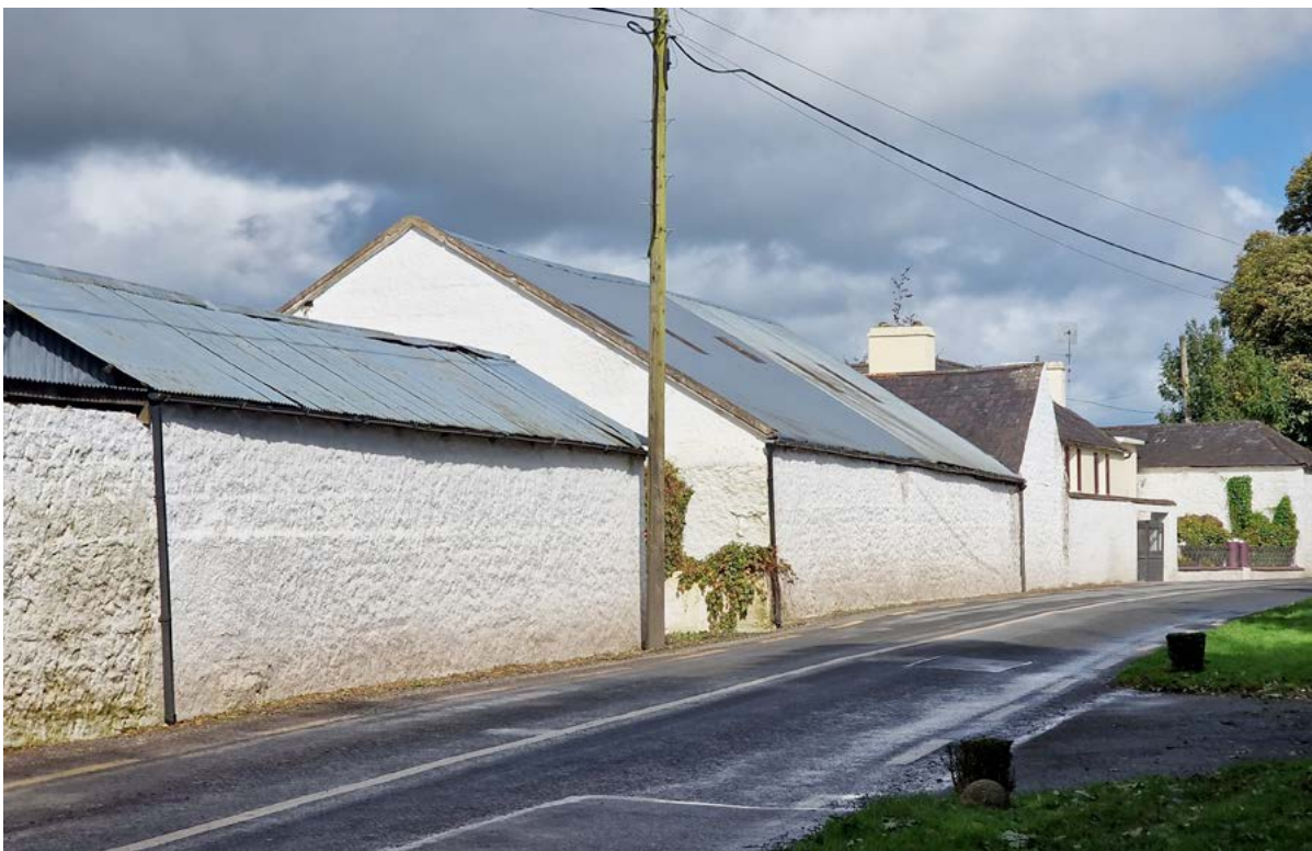
Figure 12: Limewash on traditional farm buildings
