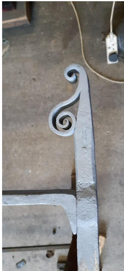
The stages in replacing the large scroll on the closing post. A new scroll is forged then brazed in the place of the old scroll using a gas torch. The brazed joint is then cleaned down and zinc phosphate primer brushed onto the bare metal.
