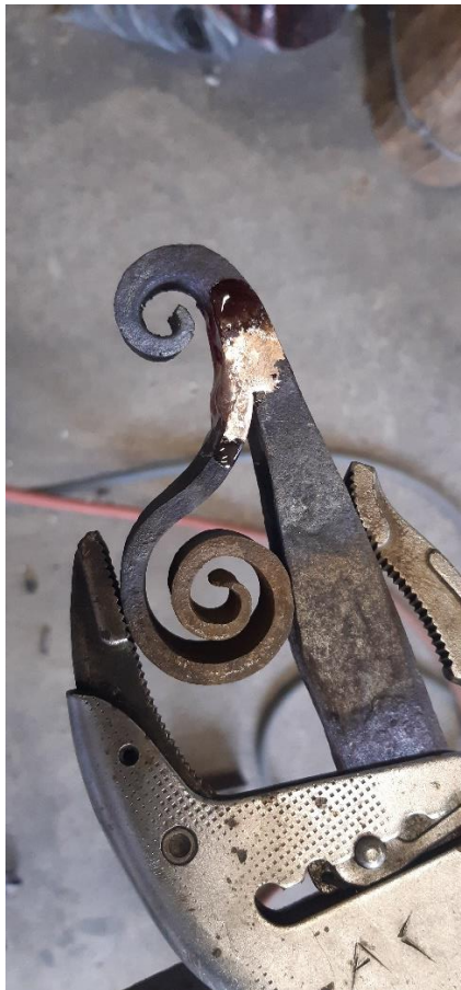
The stages in replacing the large scroll on the closing post. A new scroll is forged then brazed in the place of the old scroll using a gas torch. The brazed joint is then cleaned down and zinc phosphate primer brushed onto the bare metal.
