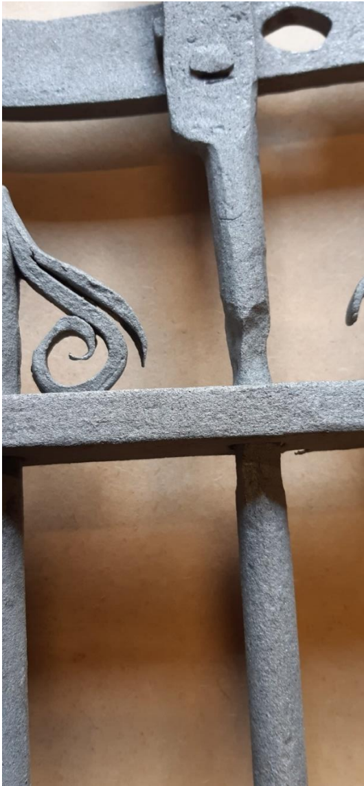
Corrosion thinning on some of the uprights
