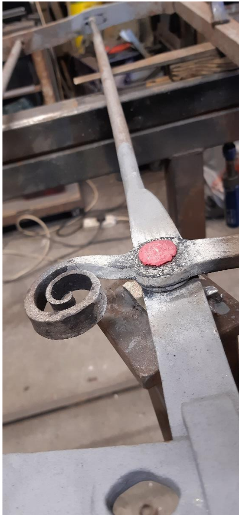
A new rivet was made and installed to replace the old worn one on the latch
