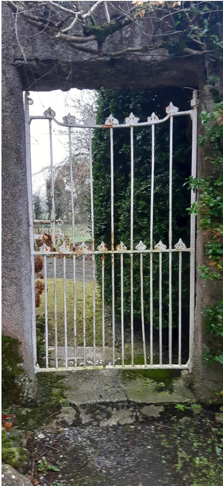
The gate prior to removal.
