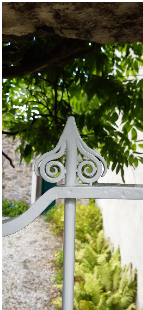
Close up photographs of the installed gate
