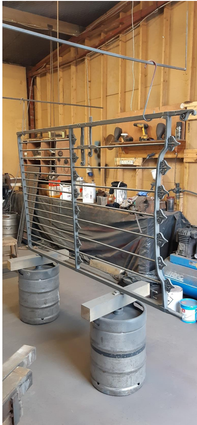
First coat of primer applied
