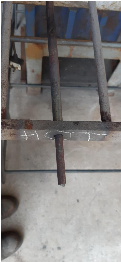
A new tenon was forged and installed to replace the broken one
