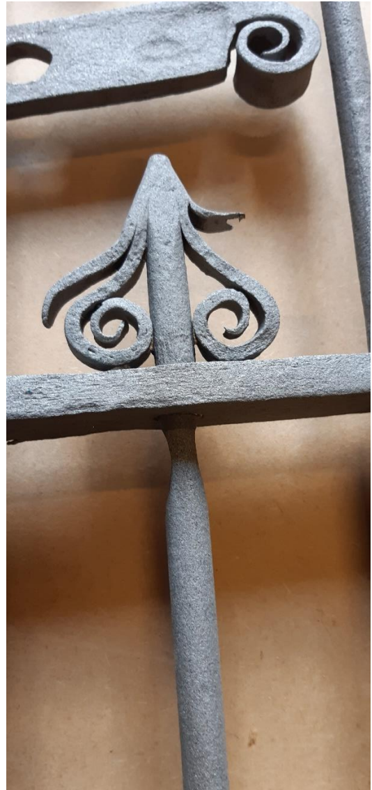
Corrosion thinning on some of the uprights
