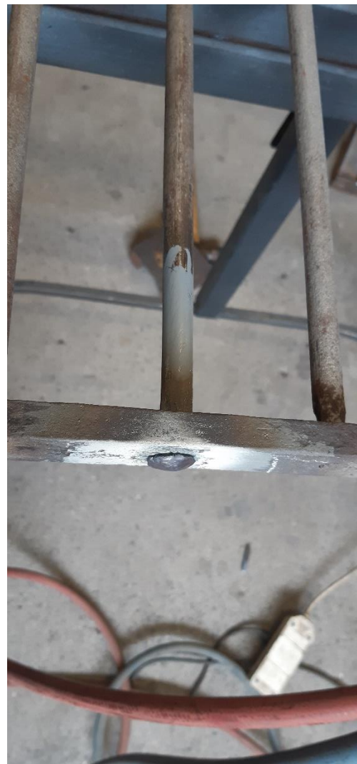
A new tenon was forged and installed to replace the broken one
