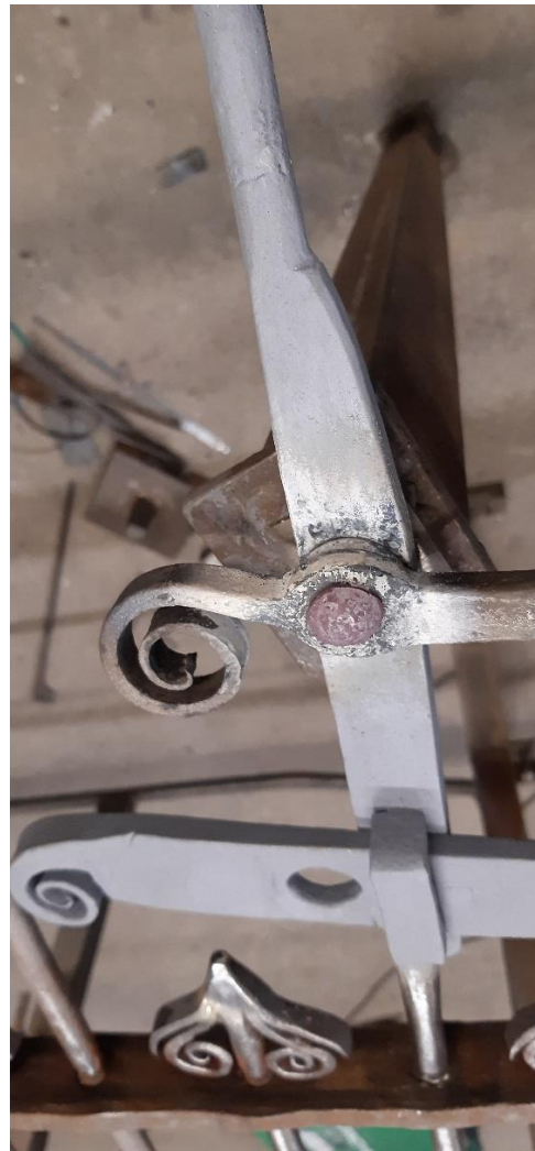
A new rivet was made and installed to replace the old worn one on the latch
