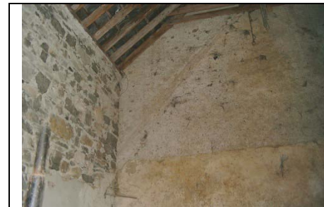
Outbuildings – internal view indicating original roof line
