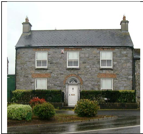
Detached House (Protected)
