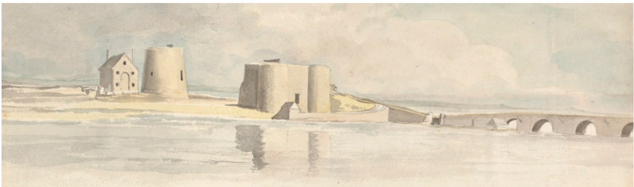
Fig. 8: View of the fortifications and (old) bridge at Banagher as seen from the Sod Battery. Drawn by Captain Sir William Smith 1819. (T.C.D., MS 942/2/187)
