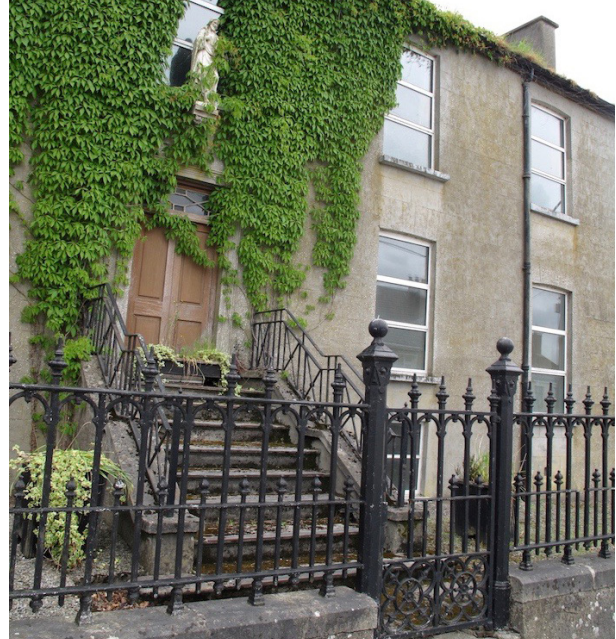
Fig. 46: La Sainte Union Boarding and Day School - Main Street entrance
