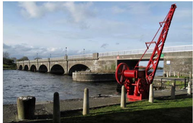
Fig. 102: Photograph of modified swivel arch, quay & Hand Wharf Crane
