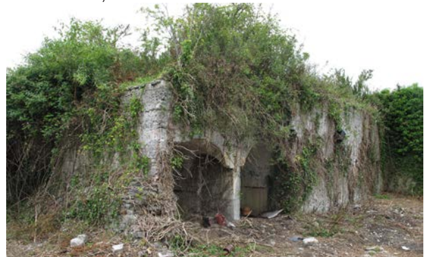
Fig. 128: Photograph of ruined magazine at Banagher Military Barracks with extensive overgrowth to the roof and former gun platform
