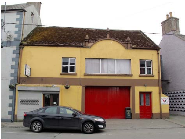
Fig. 74: Photograph of the Shannon Ballroom /Quigley's Hall
