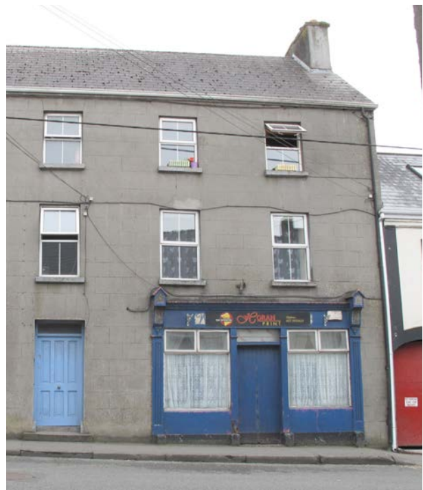
Fig. 58: Photograph of vacant traditional shopfront on Main Street
