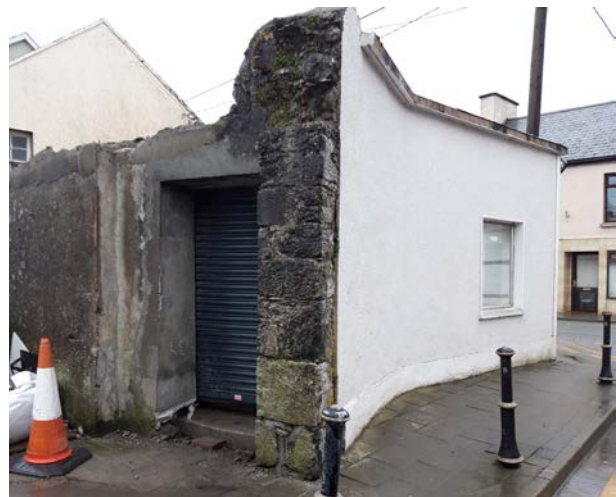
Fig. 72: Detail of 'Old Market House' south facing gable elevation, which is curiously cranked in plan with demolished integral carriage arch and hacked 'fire escape' opening to west facing elevation.
