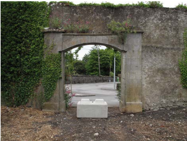
Fig. 90: Photograph of Banagher Military Barrack's entrance
