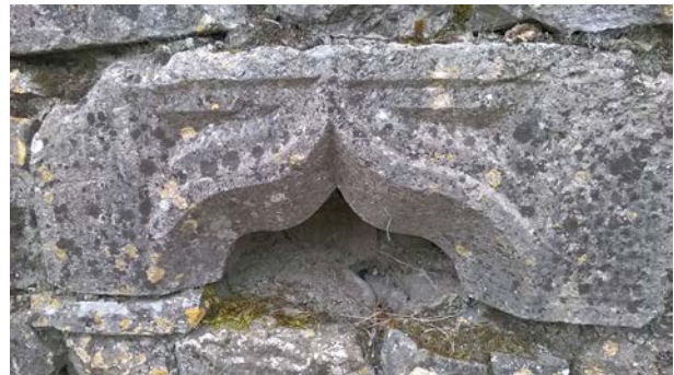
Fig. 118: Detail of fifteenth-century ogee window lintel, discovered at Banagher in 2016 (Photo by E. Broderick)
