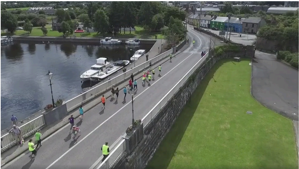
Fig. 97: Aerial photograph of Banagher Bridge ramp (image by iDrone.ie)
