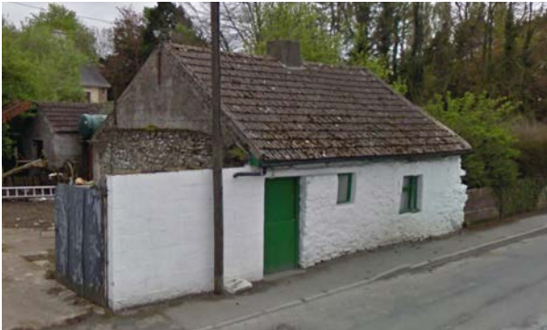
Fig. 63: Photograph of possible surviving corporation weavers' cottage on Queen Street/ Puckagh Row (image taken from Google Streetview)
