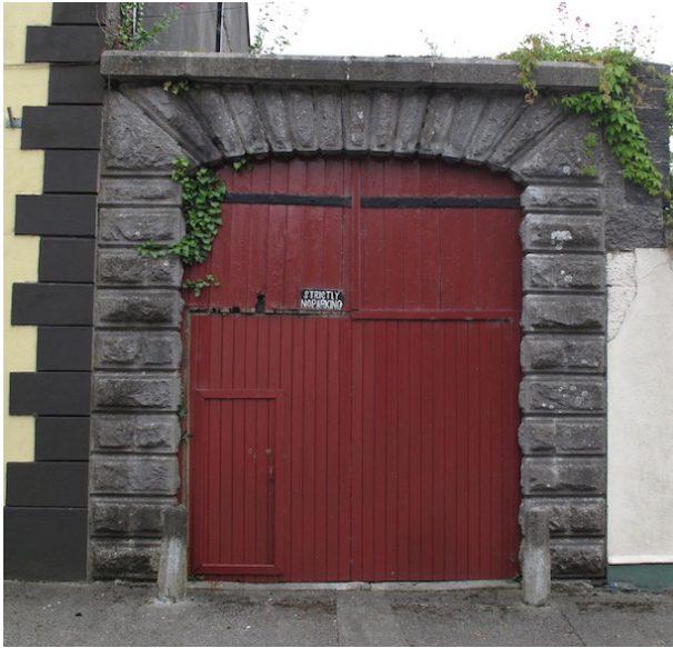
Fig. 80: Photograph of former carriage house entrance
