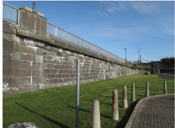
Fig. 96: Photograph of the west facing elevation of the bridge ramp
