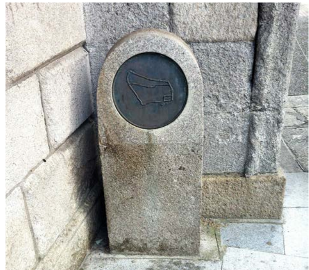
Fig. 130: Example of map of wall route (Medieval Dublin) as wayfinding street signage, consisting of bronze signplate set in cut granite pillar
