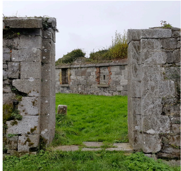
Fig. 105: Photograph of fort entrance and location of former draw-bridge
