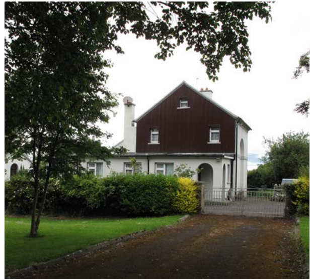
Fig. 116: View of Lock Keeper's House with modern additions (south facing elevation)
