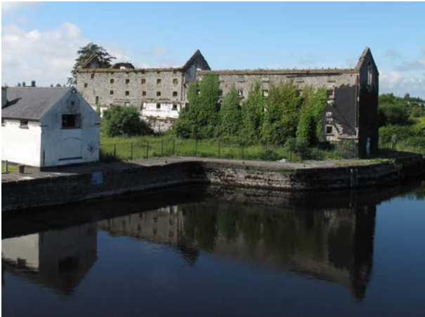
Fig. 93: Photograph of Bridge Malt House
