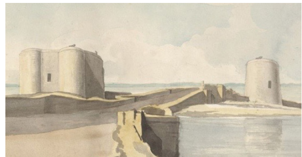
Fig. 119: View of the fortifications and Banagher's Old Bridge as seen from the Sod Battery. Drawn by Captain Sir William Smith 1819. (T.C.D., MS 942/2/187)
