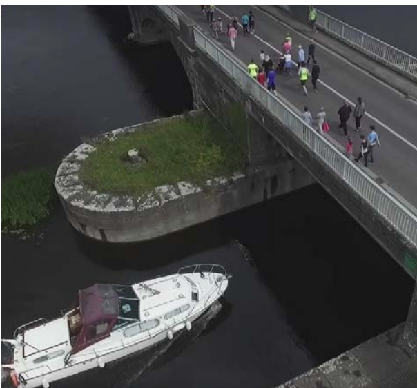
Fig. 101: Aerial Photograph of swivel arch pier (image courtesy of idrone.
