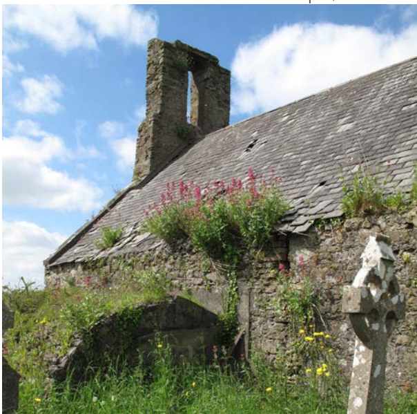
Fig. 127: Photograph of ruined late medieval Chapel of Saint Rynagh with embedded vegetation to rubble walls and eaves
