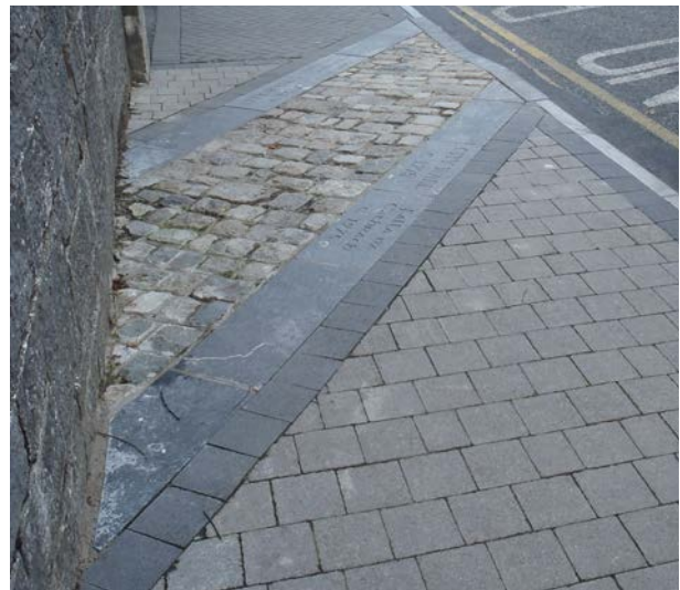
Fig. 149: Detail of paving marker indicating line of historic wall circuit in Kilkenny
