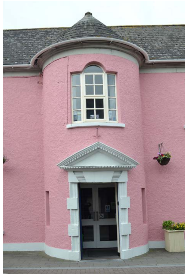
Fig. 67: Photograph of Crank House bow fronted entrance
