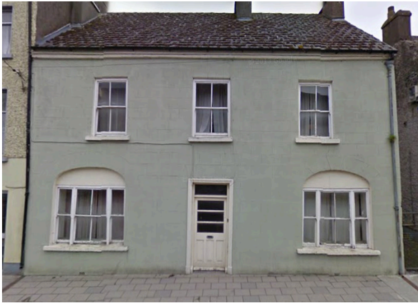
Fig. 65: Photo of Townhouse (B7) on Main Street (Google Streetview)
