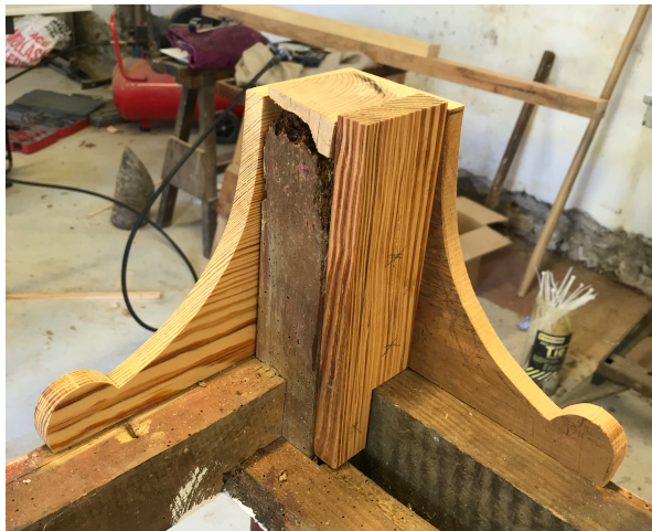
Voids filled with epoxy putty
