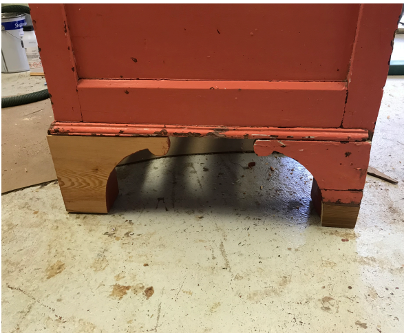
Extended back LH bracket foot
