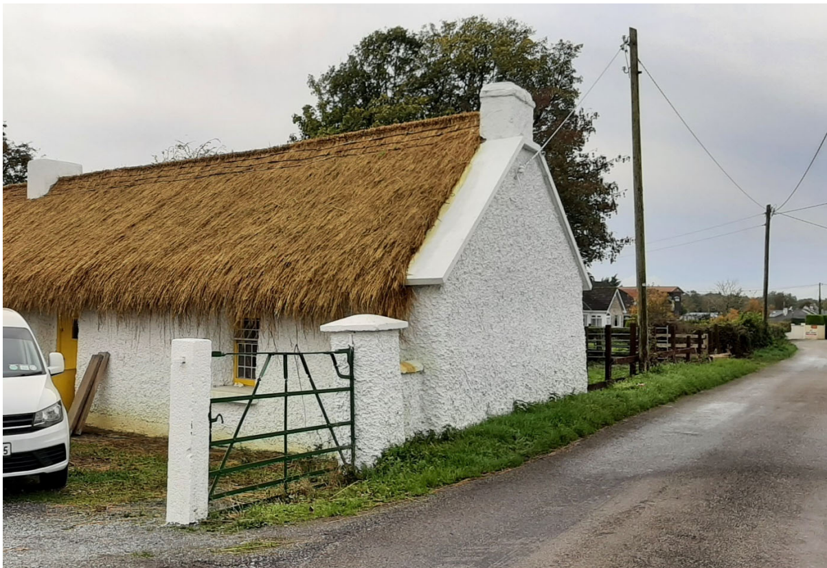
Front elevation thatching finished (eaves trimming outstanding)
