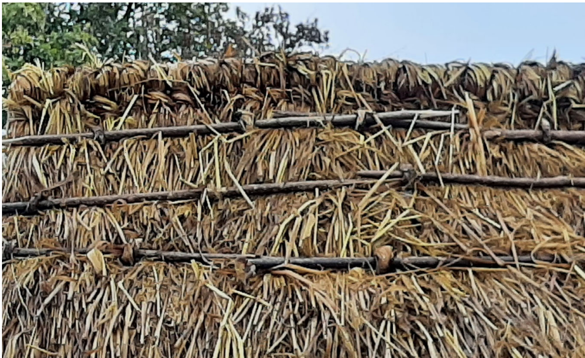
Bobbins and hazel rod detail
