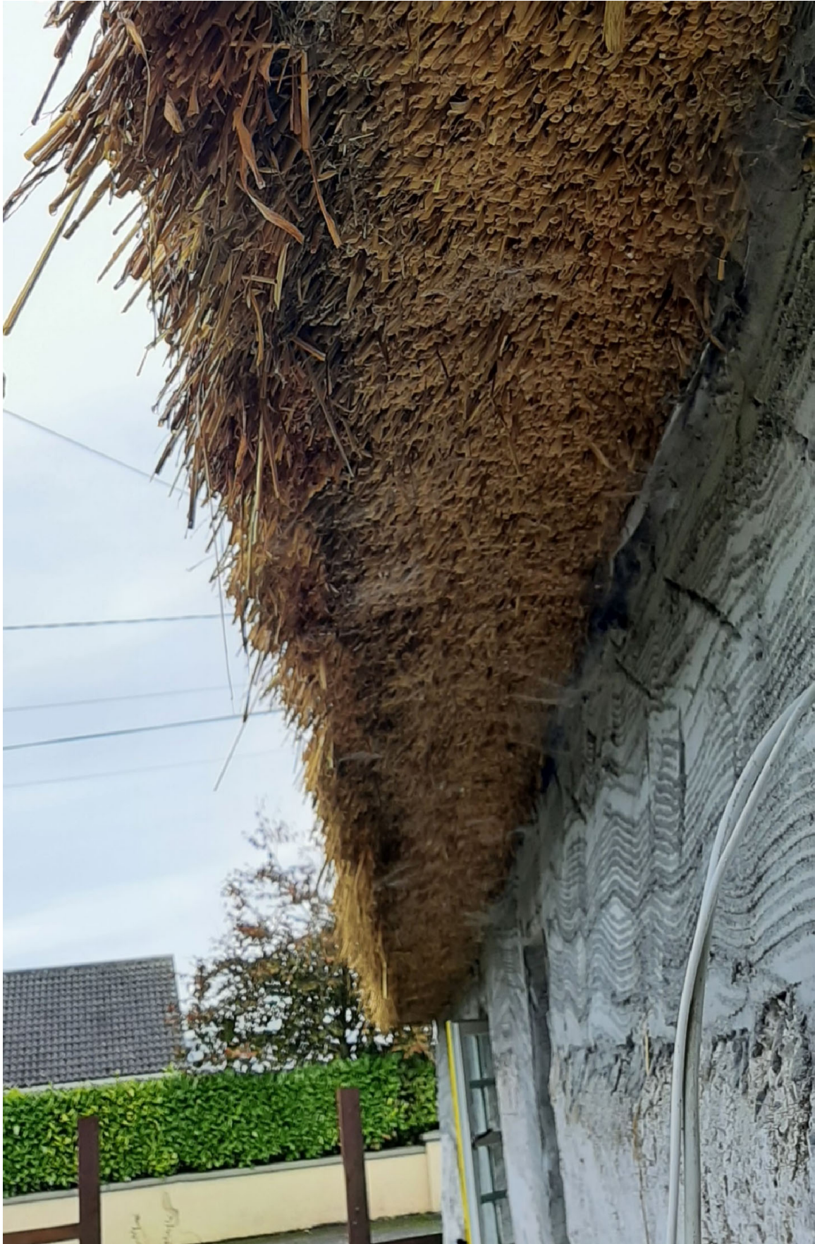
Thatch underside showing former initial layer and current new layer
