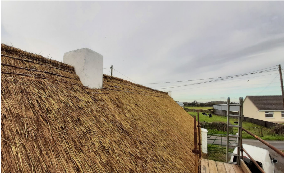
Bobbins complete tied with hazel rods
