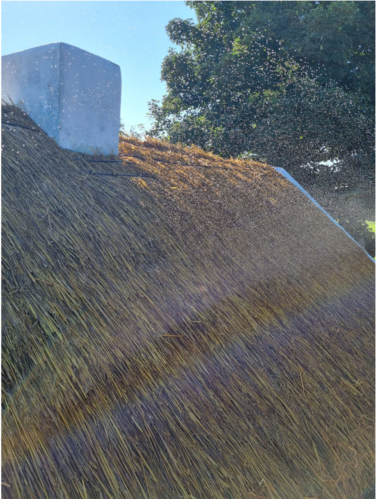
Hosing down the straw during a hot September day
