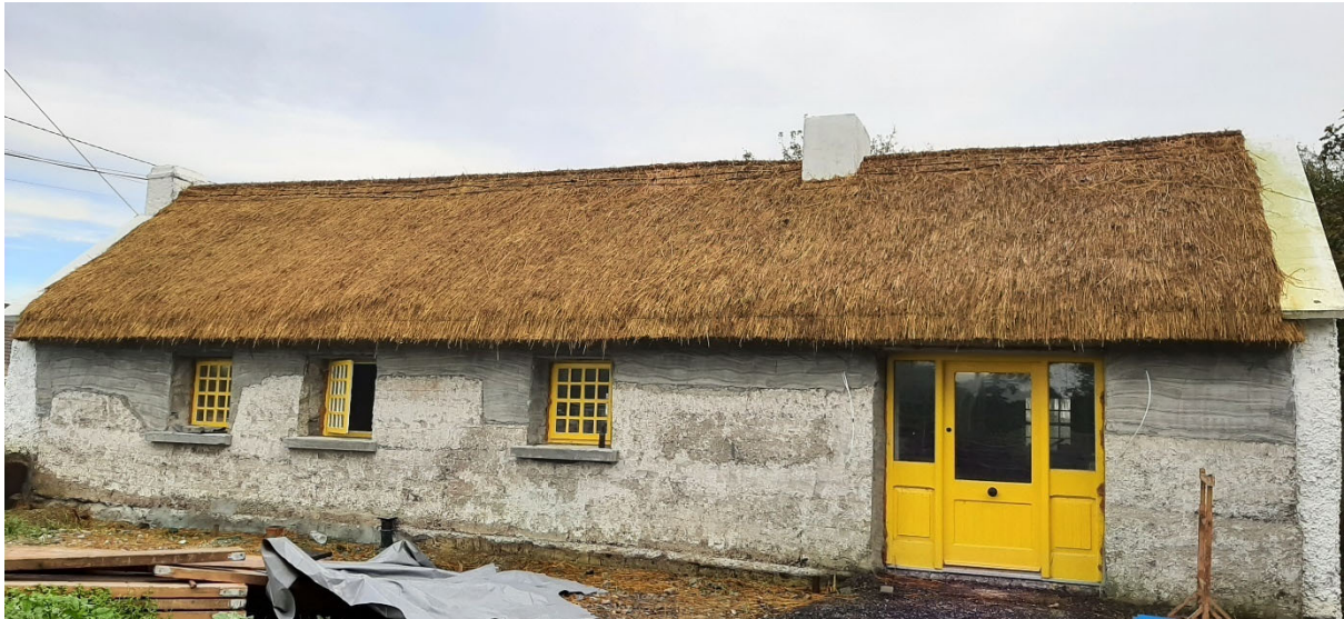
Rear complete and trimmed – October
