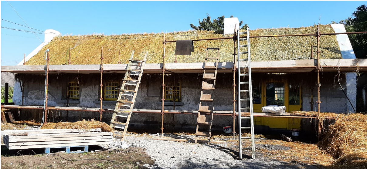
September 2023 – Works underway to the rear of the property
