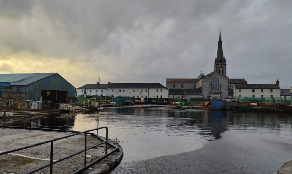
Grand Canal Harbour Site
