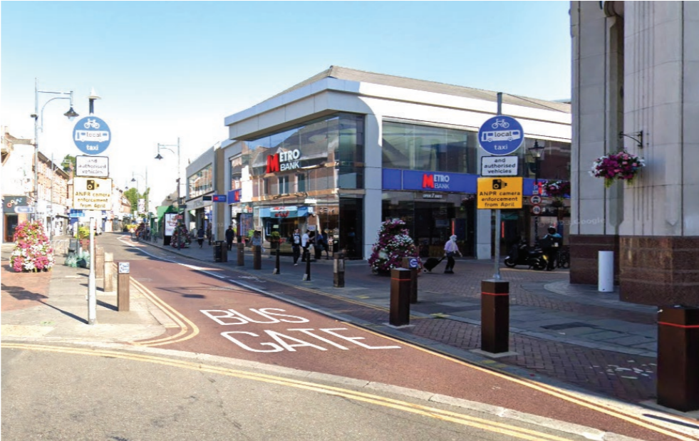
High Street, Watford, UK (east)
