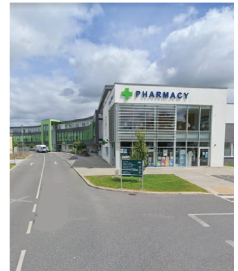
4 Primary Care Centre
