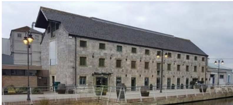
2 Former Tullamore Distillery (Protected Structure)
