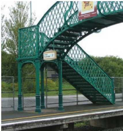
4 Railway Pedestrian Bridge
