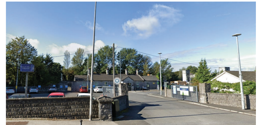
1 Tullamore Railway Station Entrance
