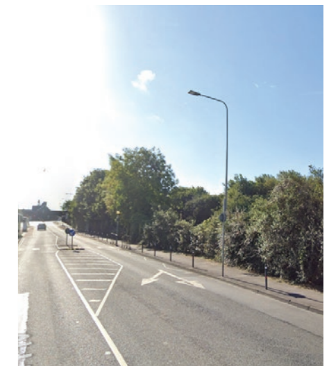
2 Main Road R433 Looking South
