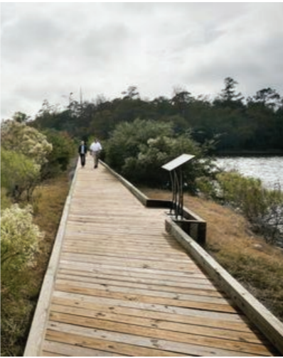
New Pedestrian Infrastructure
