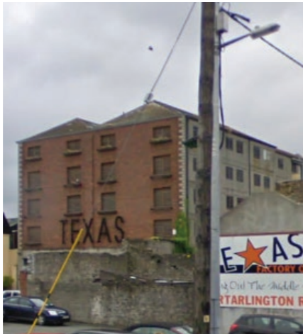
1 Former Texas Warehouse, now demolished
