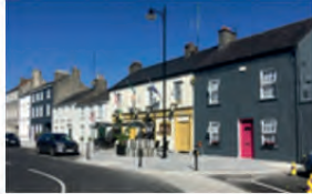
The Green, Birr – TV190Y10 Works complete, €200k claimed
