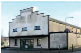
Kilcormac Enabling works complete
