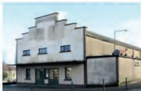
Kilcormac Enabling works complete
