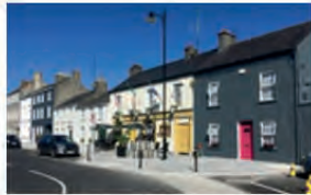
The Green, Birr – TV190Y10 Works complete, €200k claimed
