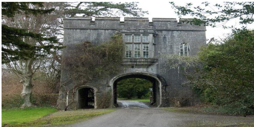
The Keep Gate, Birr – internal repairs
