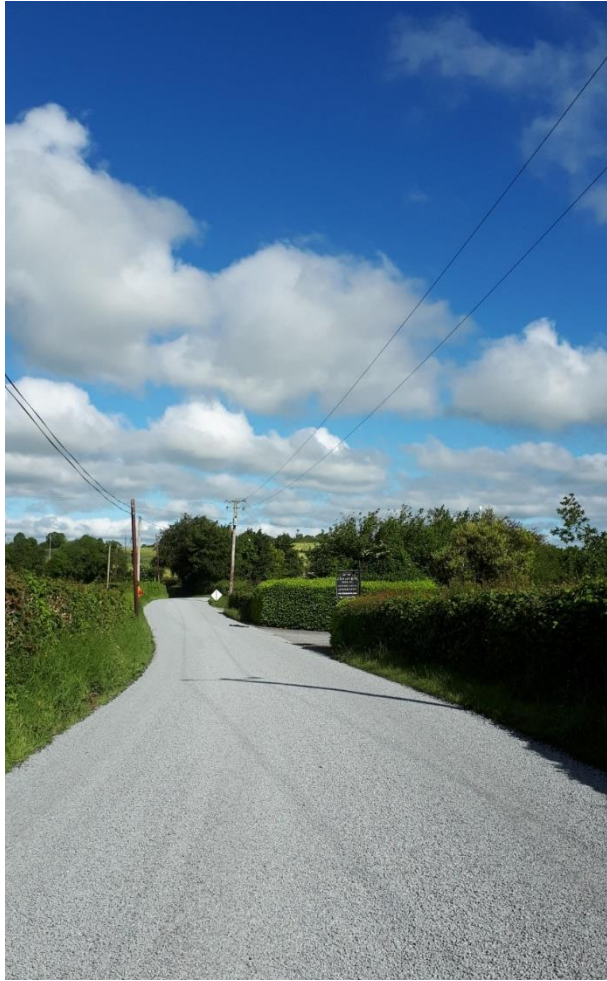
1km Surface Dressing scheme at Leap, Ballybritt
