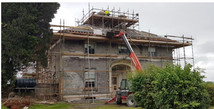
Cangort Park – roof repairs underway
