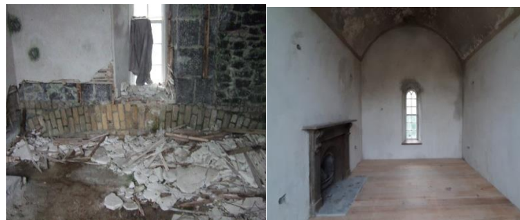
BIRR KEEP GATE – (INSIDE VIEW) BEFORE +AFTER
