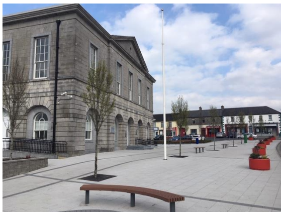
After the works – photo 2
