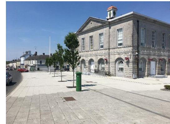
After the works – photo 1
