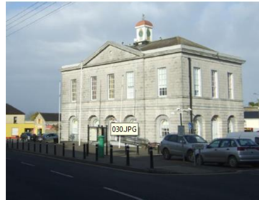
Before the works – photo 2
