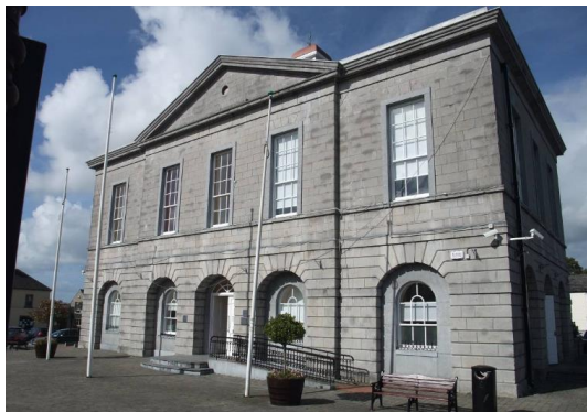
Before the works – photo 1
