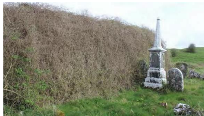
South Wall at Drumcullen Monastic Site before and after Vegetation removed
