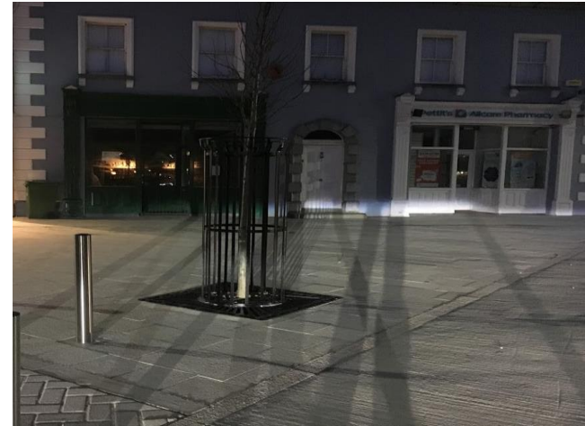
Paving works completed as part of Clara Town Renewal Scheme 2018
