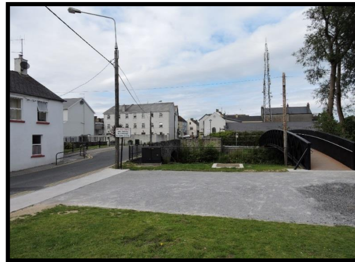
A new pedestrian Bridge was installed at Bridge Street in April 2017 as part of the Birr Active Travel programme
