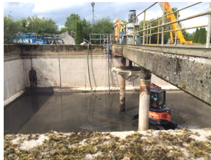
Aeration Tank Cleaning and Refurbishment Works at Birr WWTP
