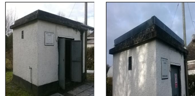
Daingean Pumping Station – Provision of New Roof
