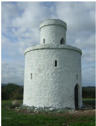
The Tower on Mullagh Hill conserved with a new coat of whitewash.
