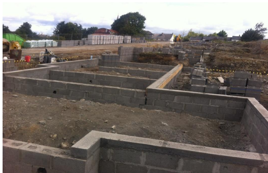
Banagher housing scheme under construction
