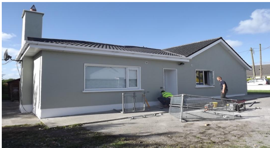
DPG Scheme underway in Edenderry
