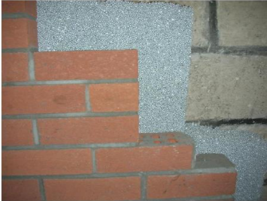
Example of cavity wall insulation
