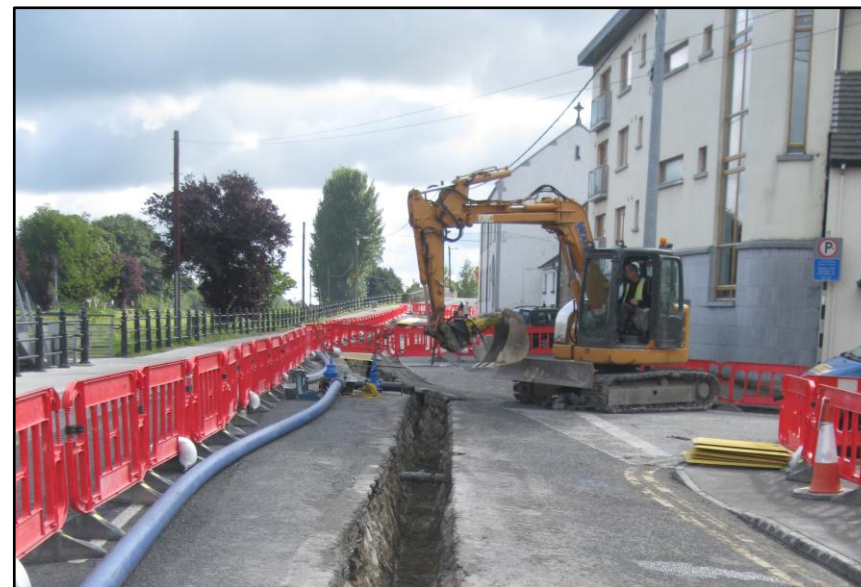
Watermain Rehabilitation Contract 1 Tullamore: New 160mm pipe on Convent Road
