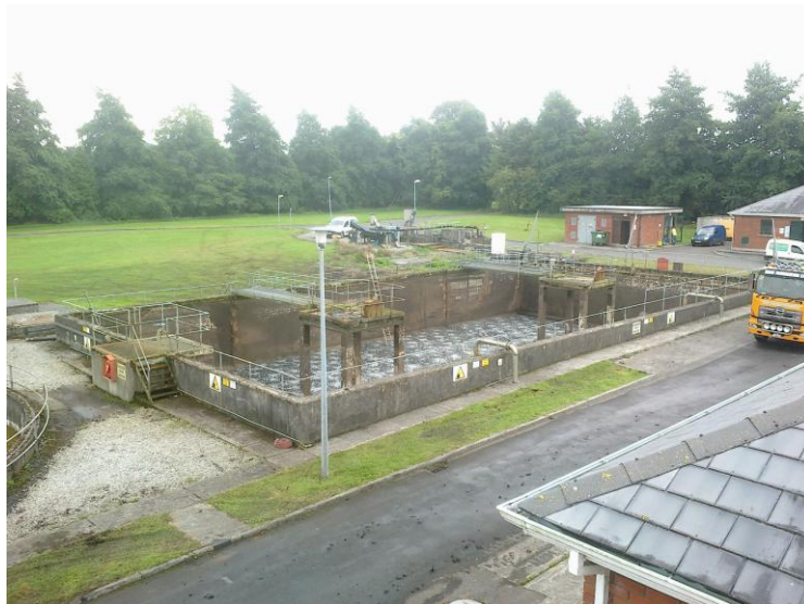
Refurbishment works at Edenderry Wastewater Treatment Works
