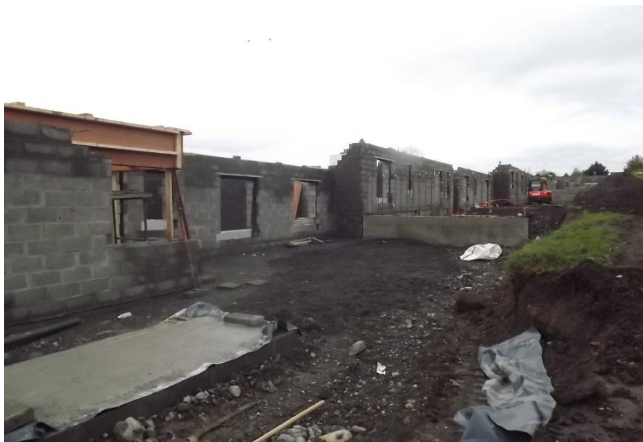
Banagher housing scheme under construction
