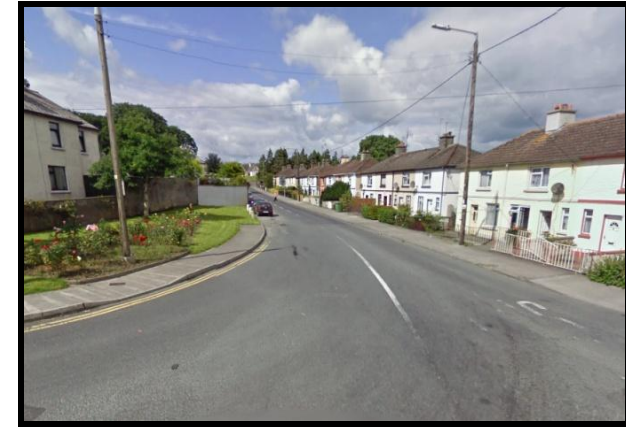
Drumbaun, Birr Before
