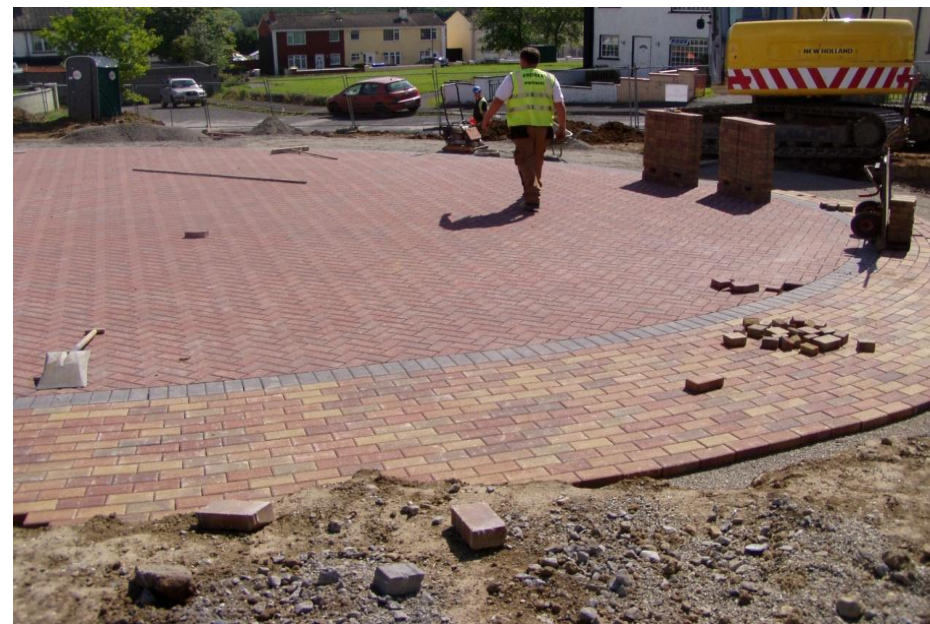
Remedial Works scheme in progress at Edenderry
