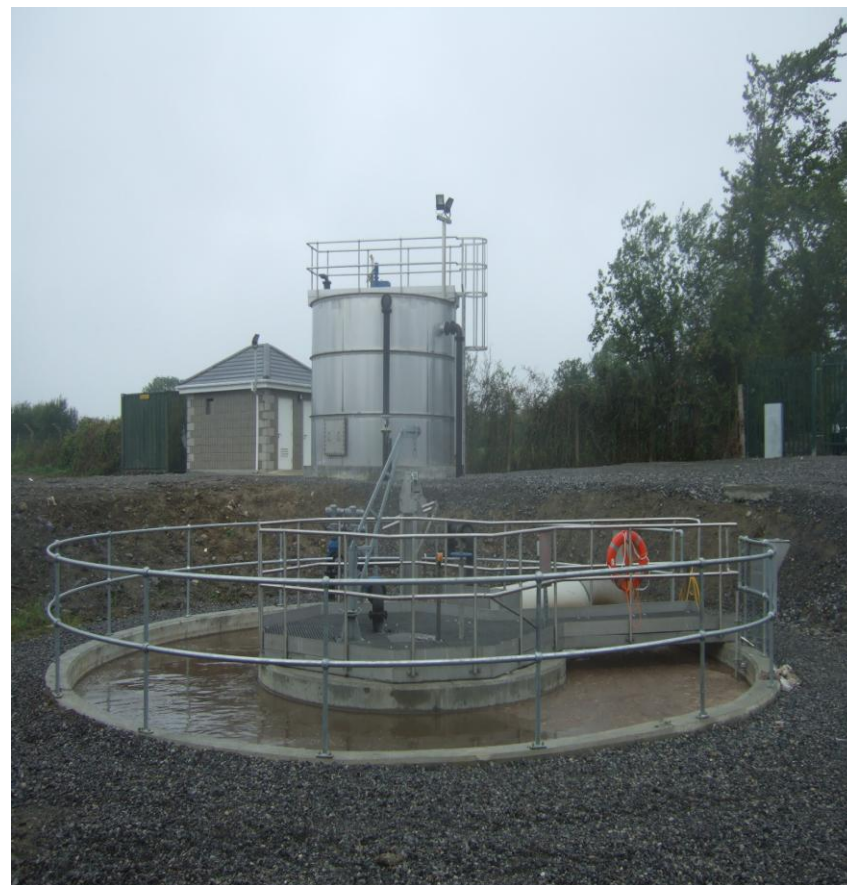
Ballinagar Wastewater Treatment Works
