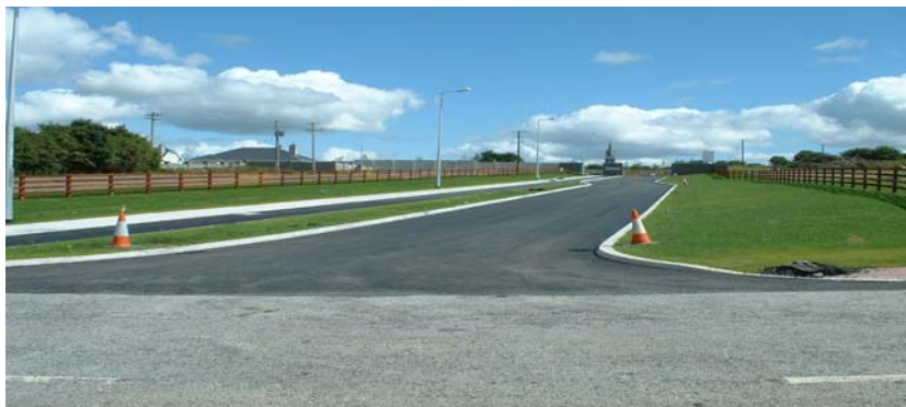
Banagher School Access Road construction
