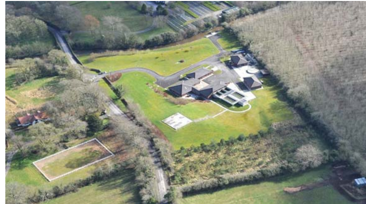
Clara Water Treatment Plant
