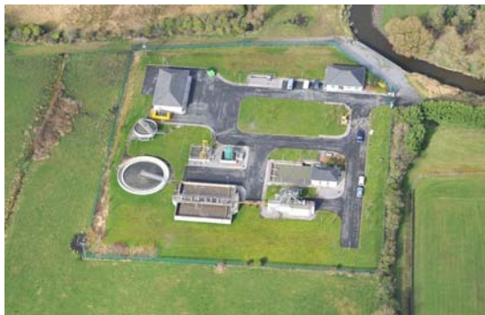
Clara Wastewater treatment plant
