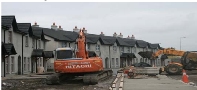
Construction activity in Cloghan
