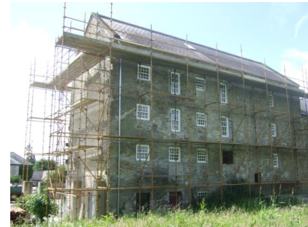
Fancroft Mill - before and during conservation works
