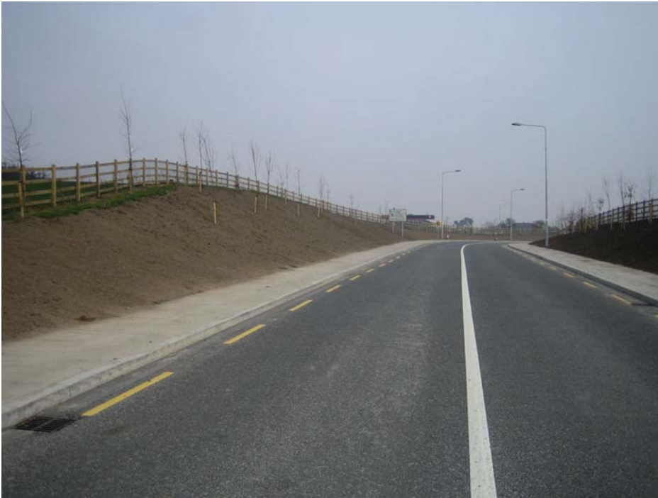
Completed - Banagher Relief Road December 2006
