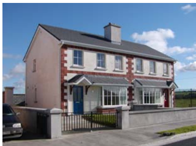
Affordable Housing under construction in Kilcormac
