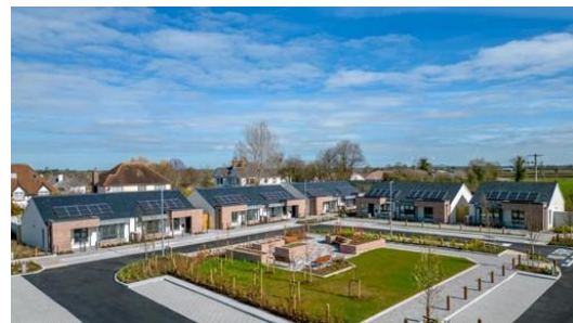
An overview of the Ashfield development.
