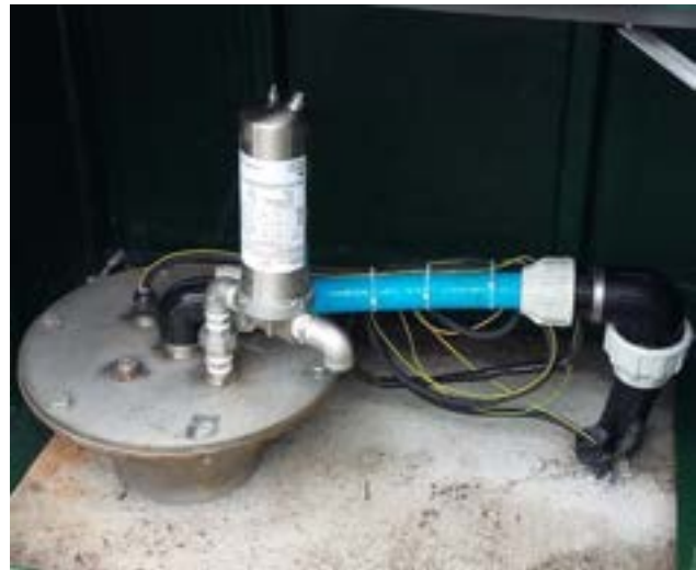
Figure 2: a properly sealed borehole
