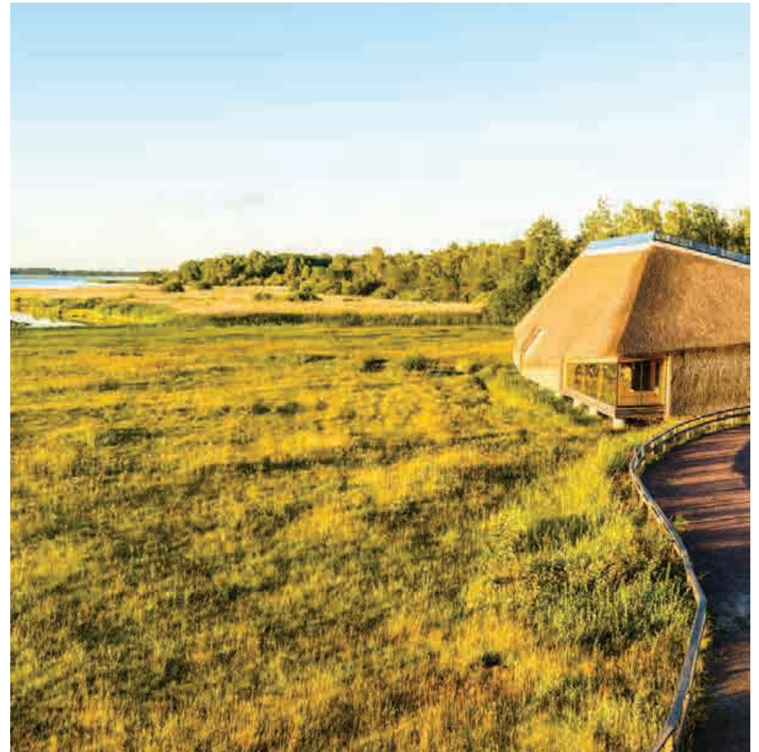
Above: Naturum Lake Tåkern sits on piles at the edge of the lakeshore wetland and the surrounding pine and spruce forest. Reed-thatched roofs slope steeply down to the building's raft floor, with large windows cut into the walls to enjoy specific views over the habitats.
