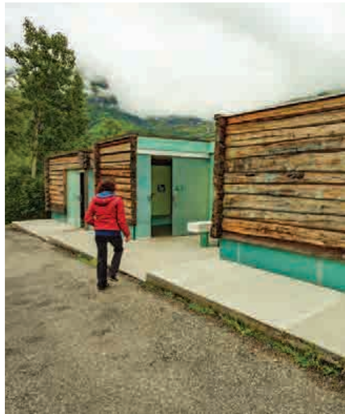
Above: precedent image of one of the rest facilities provided for tourists along the Norwegian scenic route
