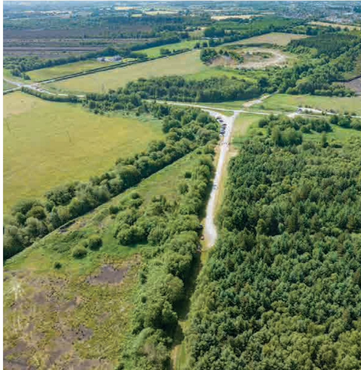
Above: aerial photograph of the Derryvilla entrance
