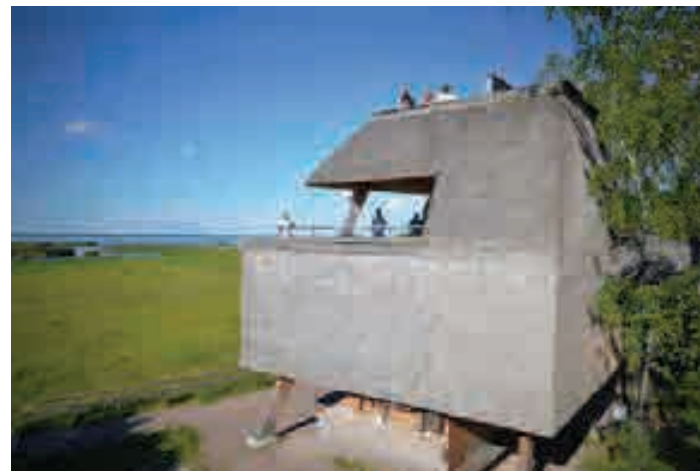
Above: Overhanging roofs cantilever over open spaces to allow visitors to shelter in all weathers at Naturum Lake Tåkern, Sweden.
