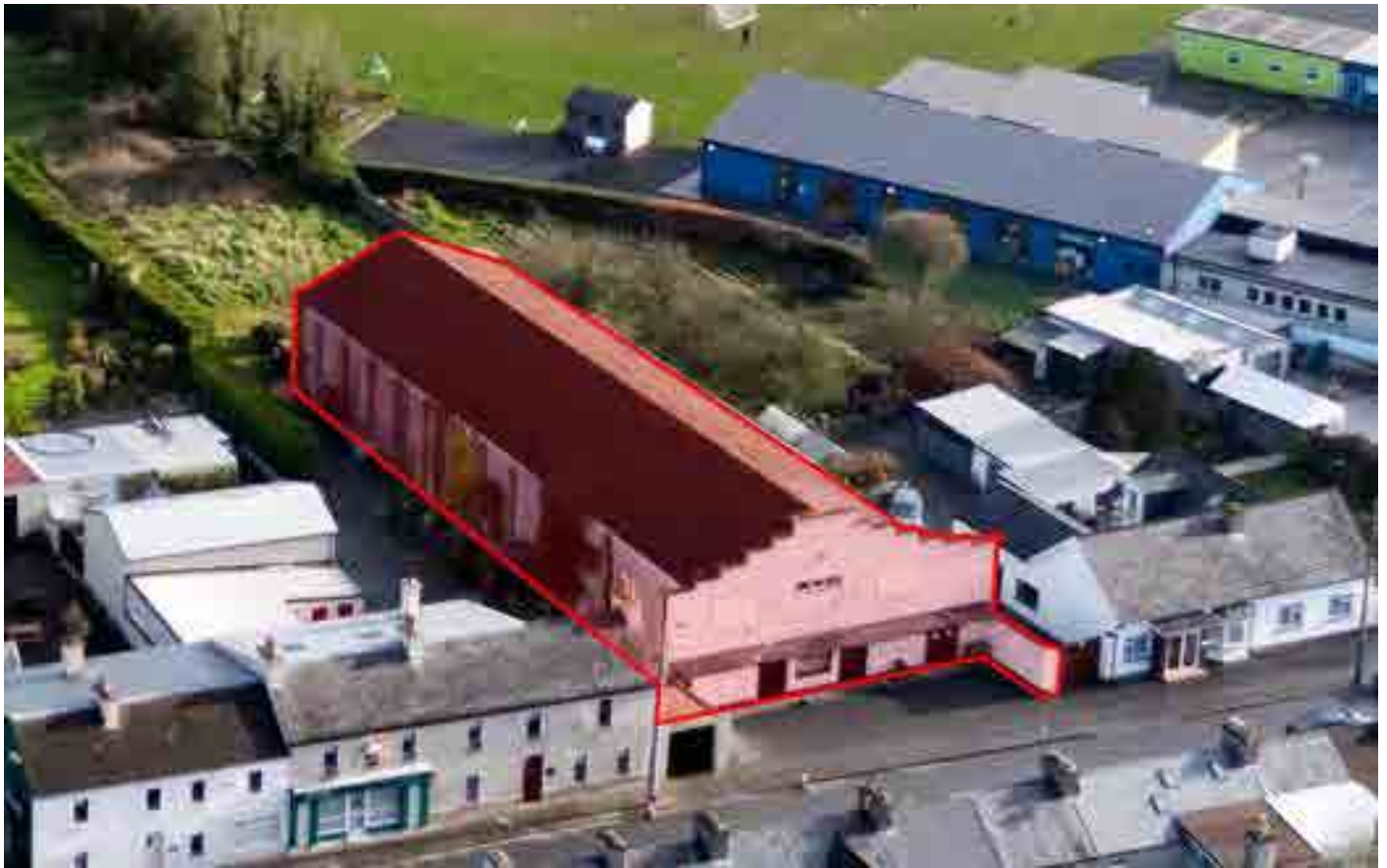
Figure 4.14 Location of the Star community hall on River Street (Aerial View)
