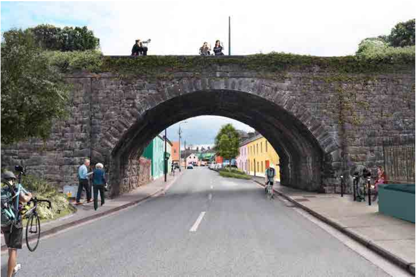
Figure 4.18 Future Railway Greenway link on River Street
