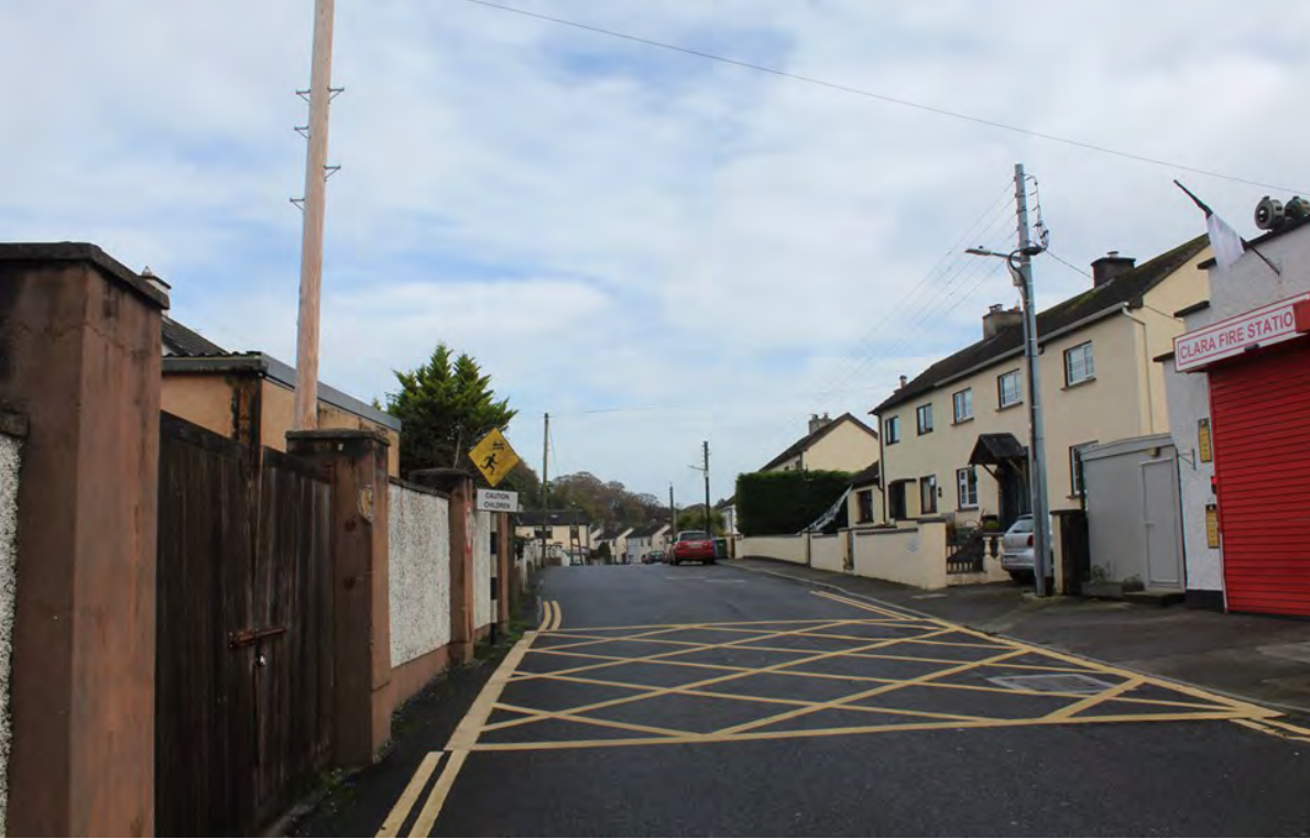
River Street (ground level difference between footpath and carriageway)
