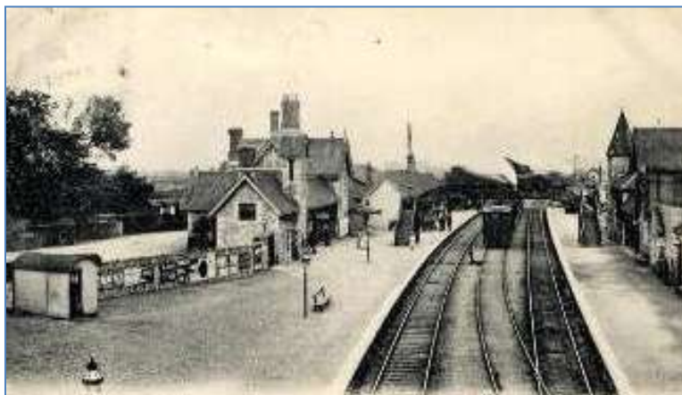
Figure 21: Portarlinton Railway Station 1950
