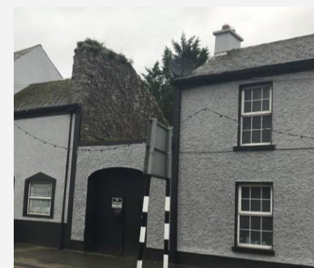
Figure 8. Exposed masonry on French Church Street
