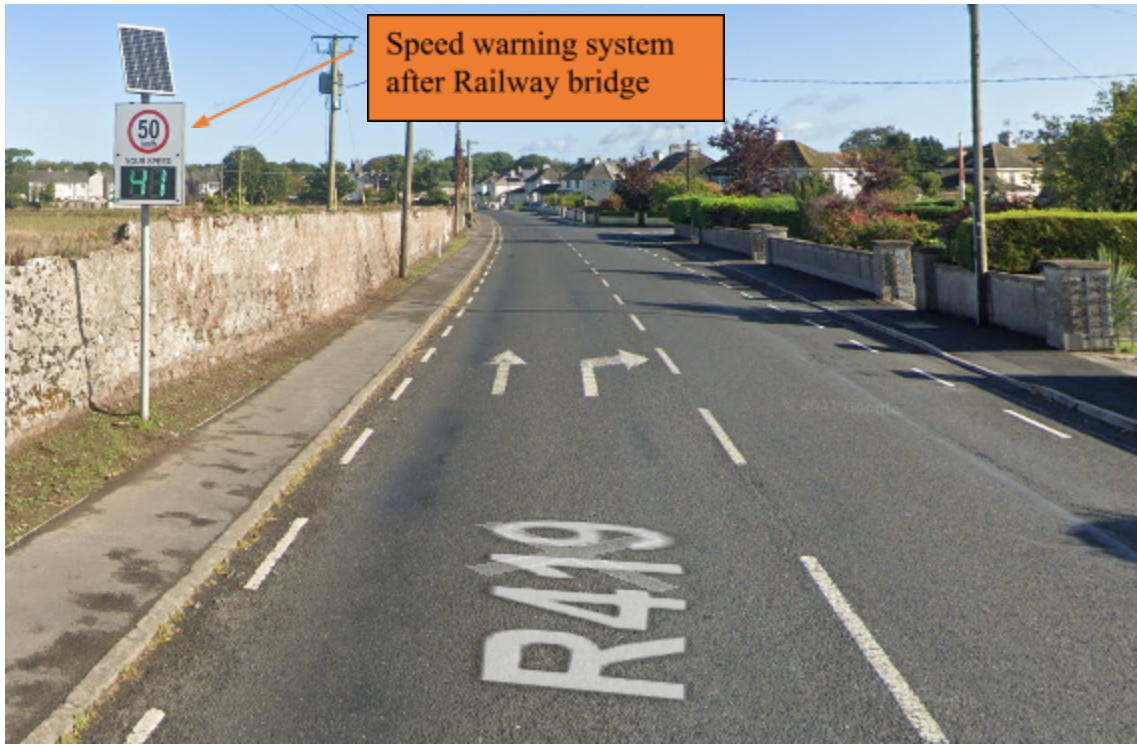
50kmh speed limit at Railway Bridge inbound
