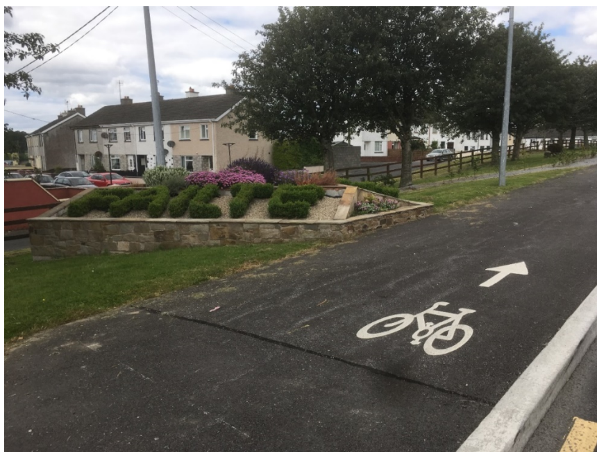
Figure 7.3 Cycleway in Gallen on southern entrance to town
