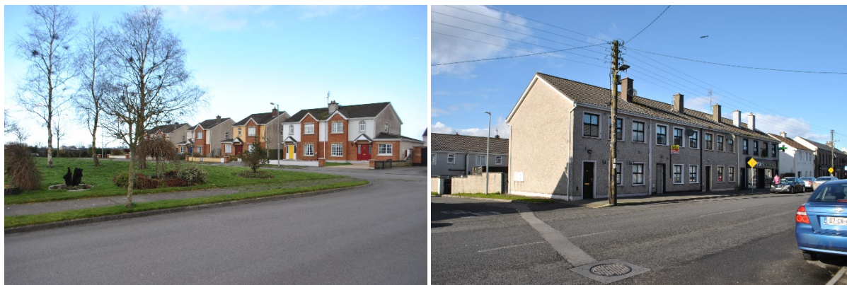
Figure 2.6 Existing Residential Development in Daingean
