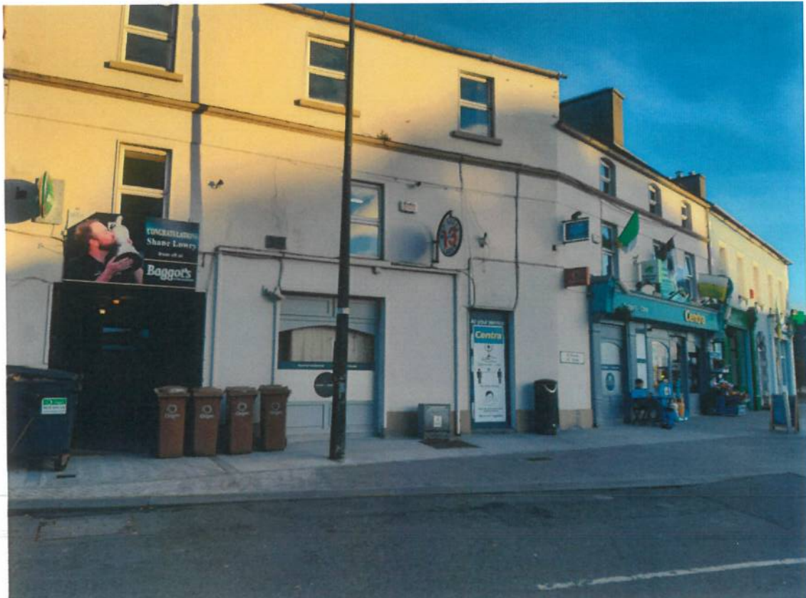
Plate 1: View of entrance to alleyway way to access public house
