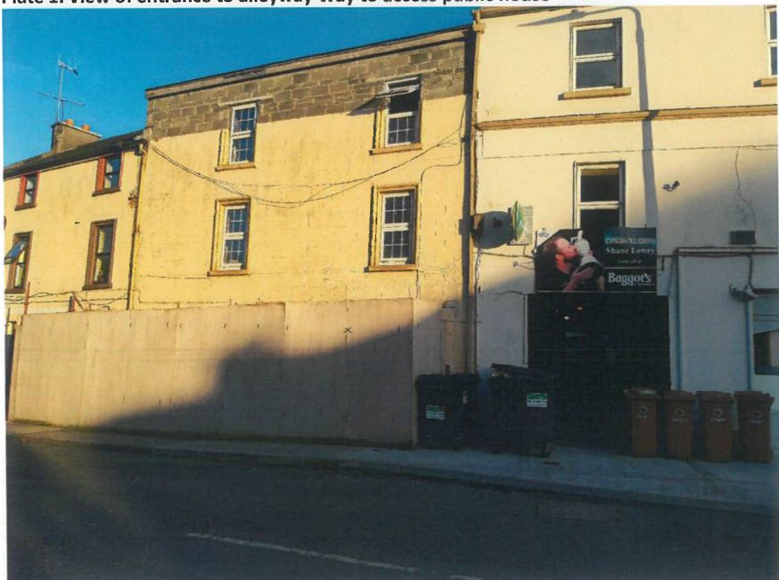
Plate 2: view of adjoining building to the north (outside landholding)
