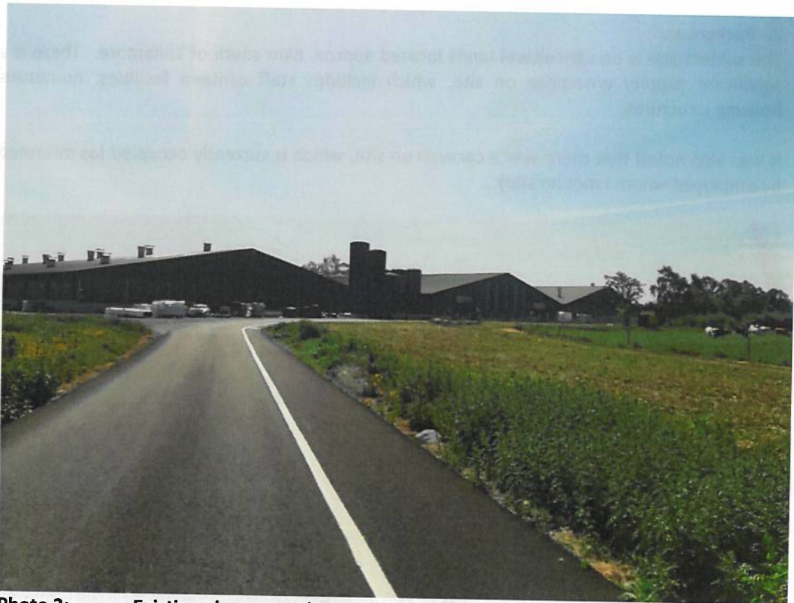
Photo 2: Existing piggery on site
