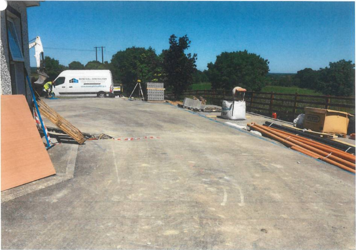
Works underway at the west elevation.
