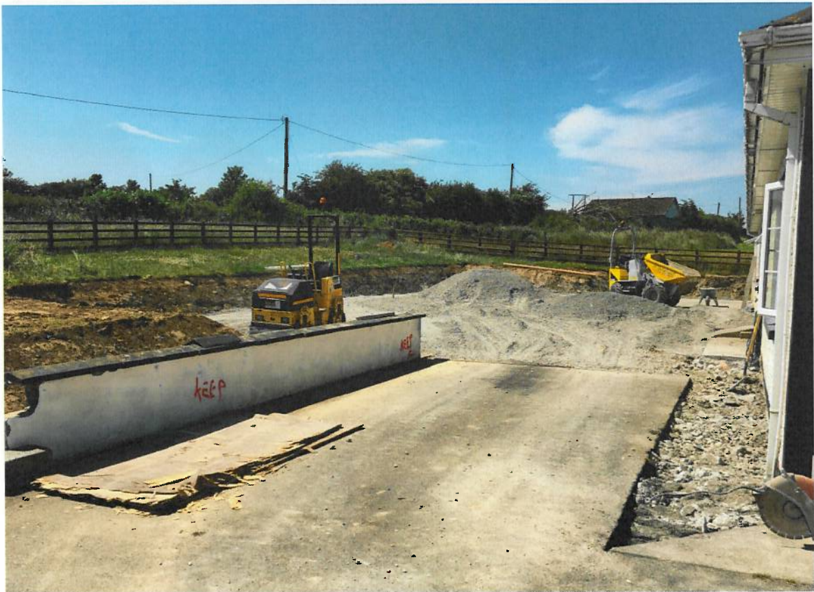
Works to the rear of dwelling (individual gardens to be created)
