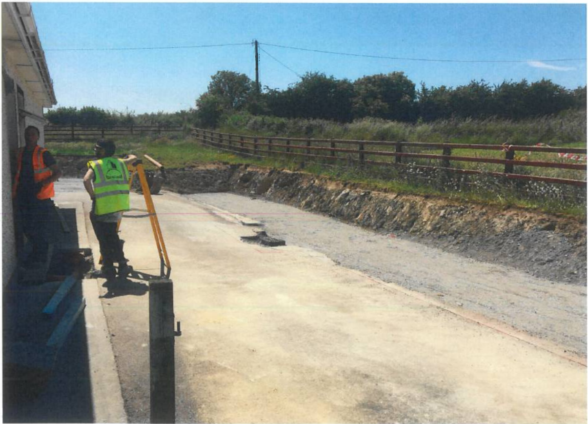
Works underway at the east elevation.
