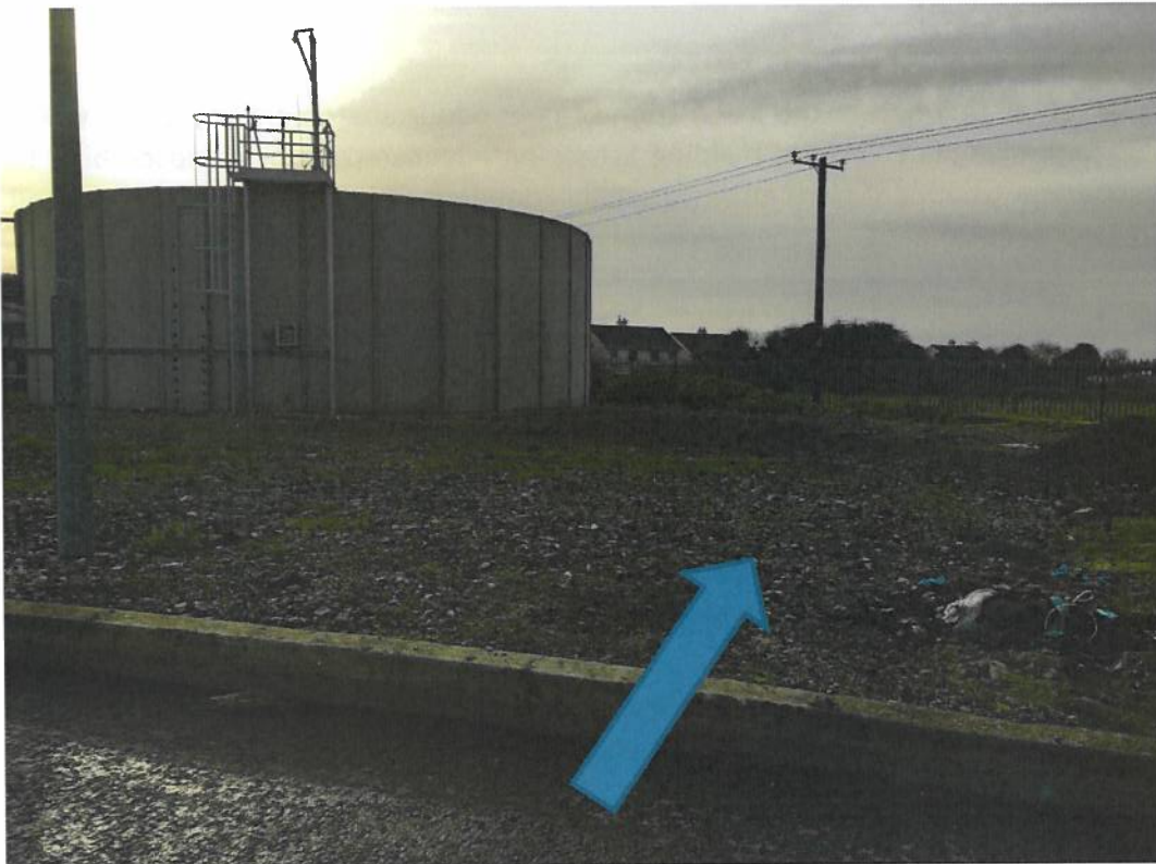
Photo 2: Location of Aeration Tank adjacent to existing Tank.
