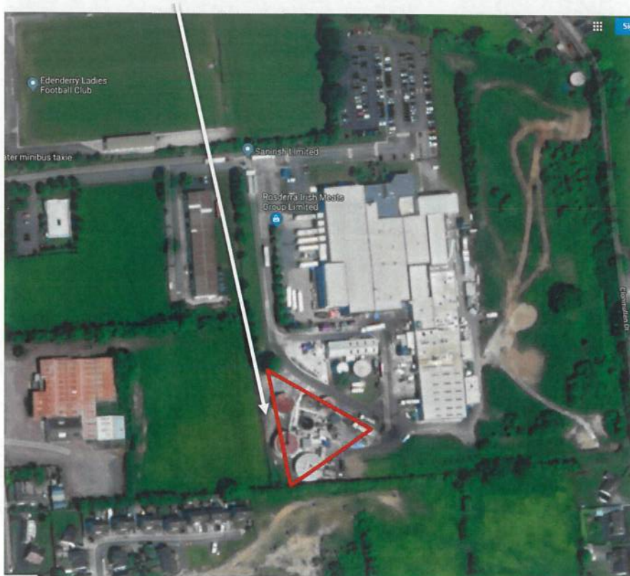
Photo 1- Approximate location of Proposed Aeration Tank, new sludge dewatering building, Inlet sump building, and bioscrubber.
