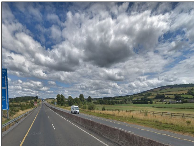
Figure 8.8 M7 Motorway in County Offaly
