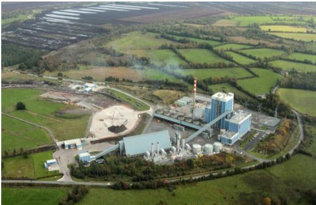
Figure 5.10 Edenderry Electricity Generating Power Station
