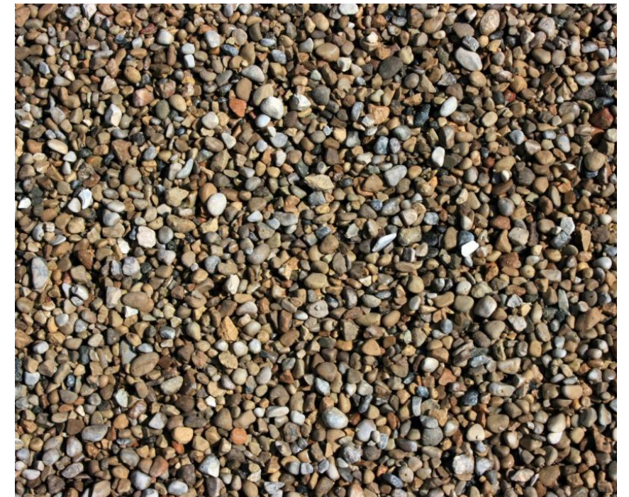
Loose Gravel to driveways
