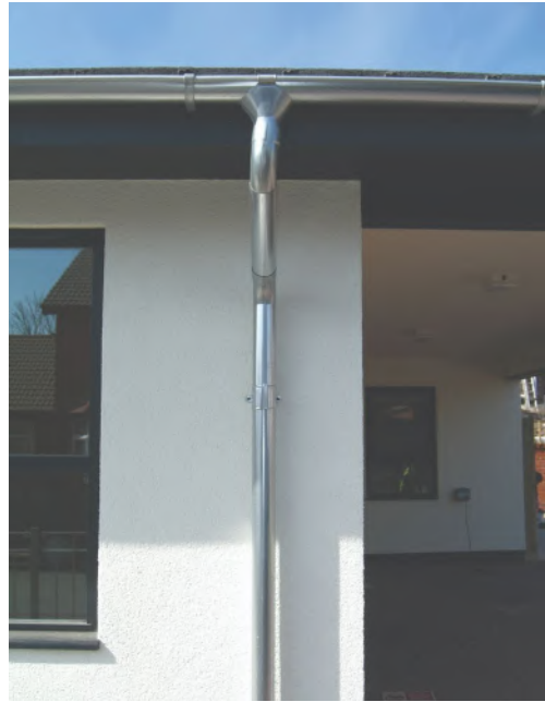
Galvanised round guttering/downpipes
