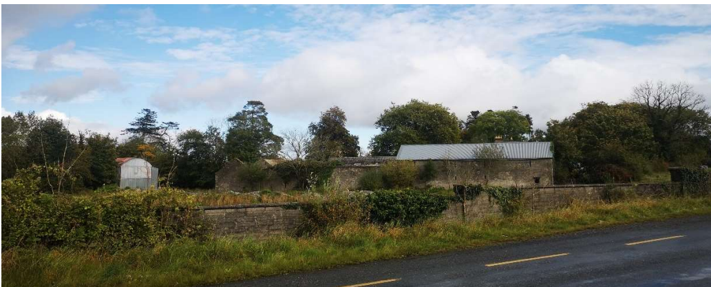
View of Development Site September 2020 (site has been cleared), (new) Portarlington Rd R401
