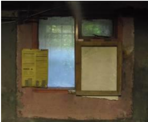
Figure 04: Basement Window in B 003
