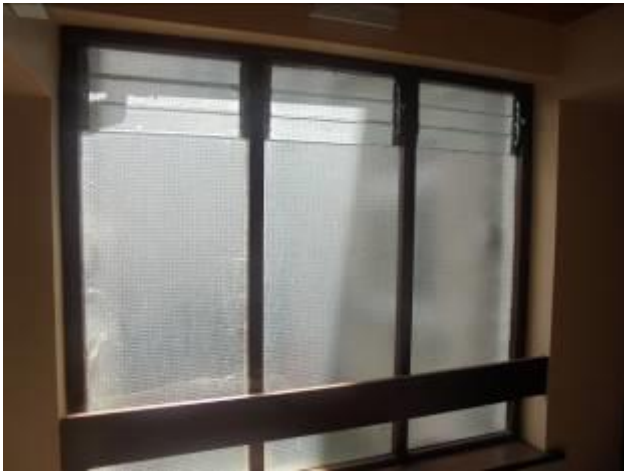
Figure 15: Window in GF 004
