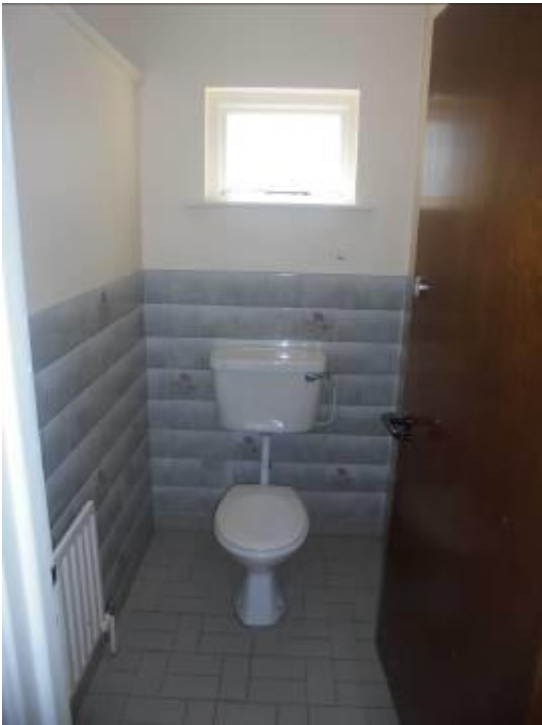
Figure 21: View of details in GF 008
