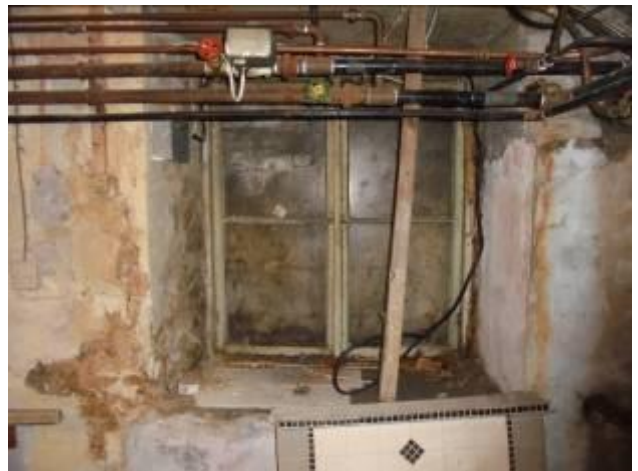
Figure 07: Basement Window (sealed) in B 004
