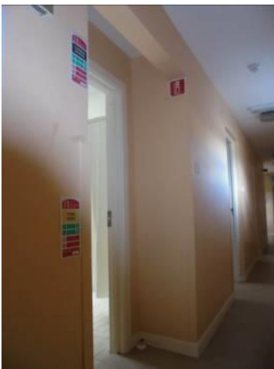
Figure 25: View of Beam in GF 011
