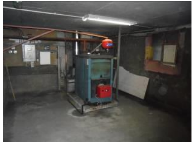
Figure 05: View of B 003
