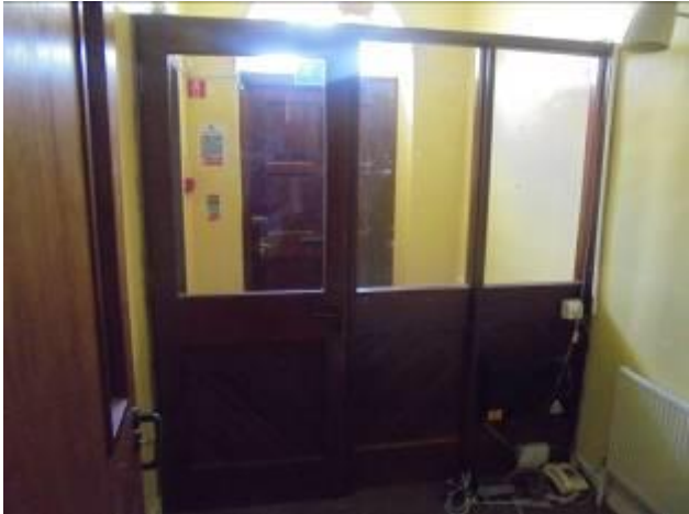
Figure 10: Partition screen in GF 001
