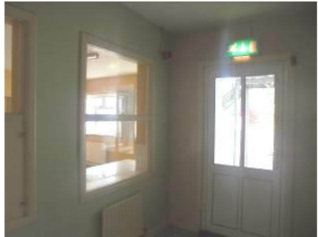
Figure 42: Lobby Room GF 022
