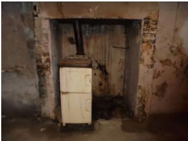
Figure 06: Existing stove in B 004
