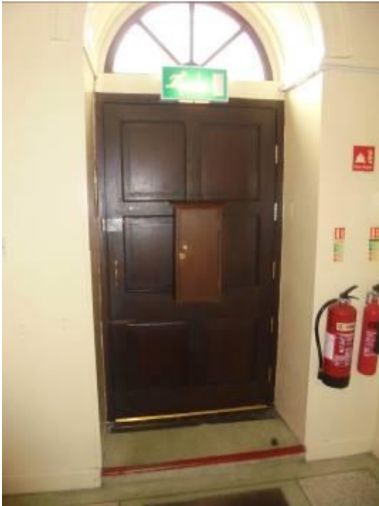
Figure 32: Detail of door at GF 017
