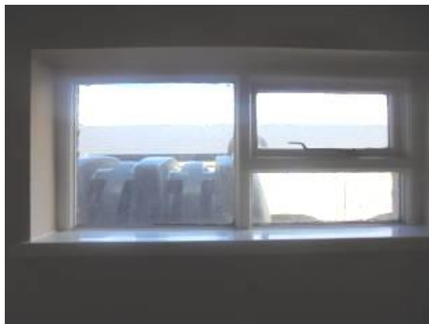
Figure 24: View of window in GF 010
