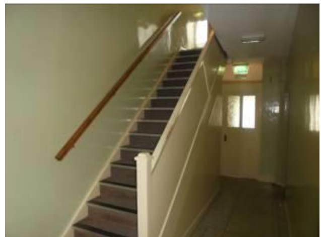
Figure 35: Stairwell in GF 018
