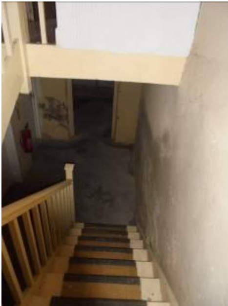
Figure 01: View from stairway landing in B 001
