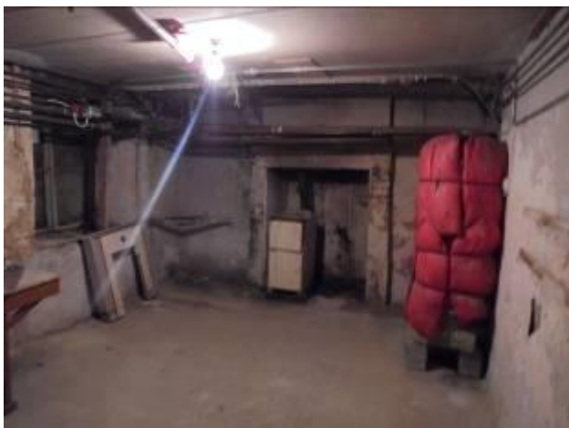
Figure 08: View of B 004
